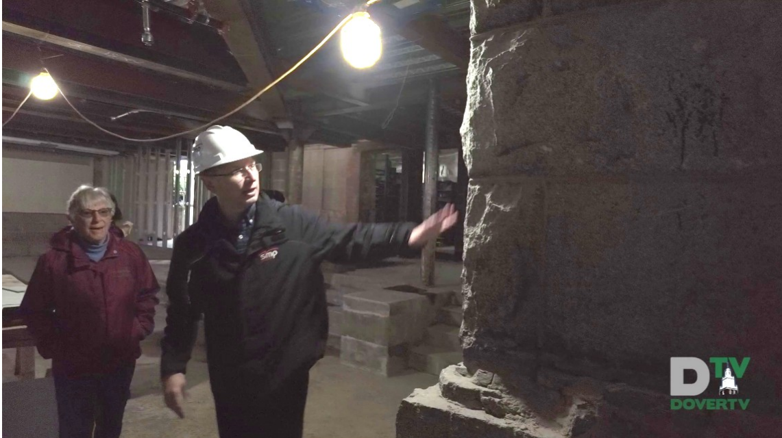
Architect Jason LaComb shows off the library's granite foundation uncovered during the project.
