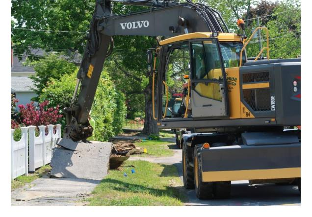
A contractor with John H. Lyman & Sons, Inc., uses an excavator to remove old sidewalk pavement on Rutland Street on Tuesday as part of a planned sidewalk reconstruction project.
