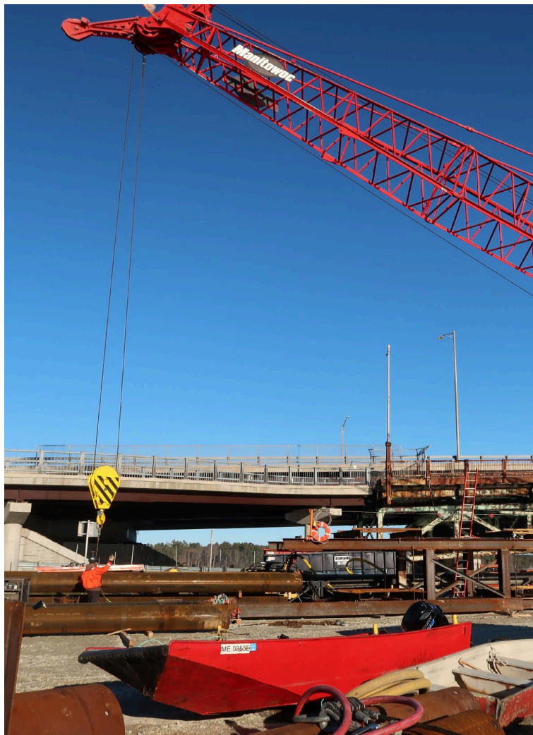
A crane begins lifting a steel column that will be used to create a temporary trestle to remove the General Sullivan Bridge.
