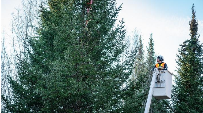
Ryan Neenan of Community Services prepares to attach a winch to a 50-foot balsam fir on Piscataqua Road before the tree is cut down and moved by crane.
