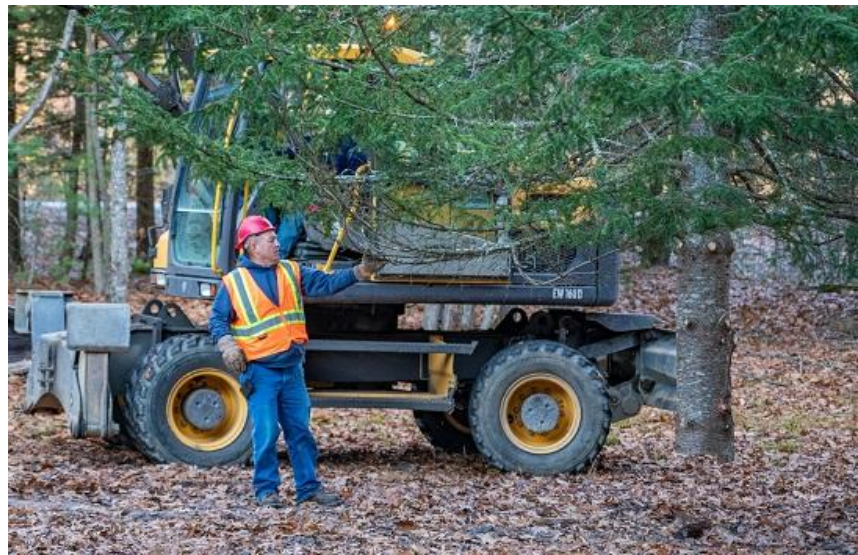
Dean Truax of Community Services helps guide a 50-foot balsam fir on Piscataqua Road after it was cut and moved by a crane.
