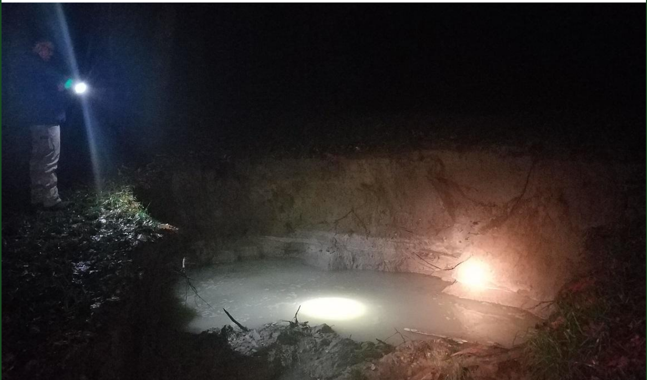
Community Services crews at the site of a significant water leak on Christmas Day.
