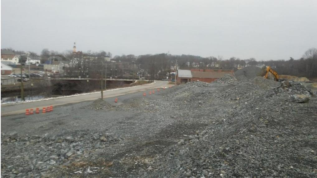
Much of the excavated material will be used to raise the elevation of the waterfront site in preparation for future building development. The remaining materials consisting of processed rock and stone dust will be used by the City to construct streets and utilities on the waterfront site as part of the site development process.
