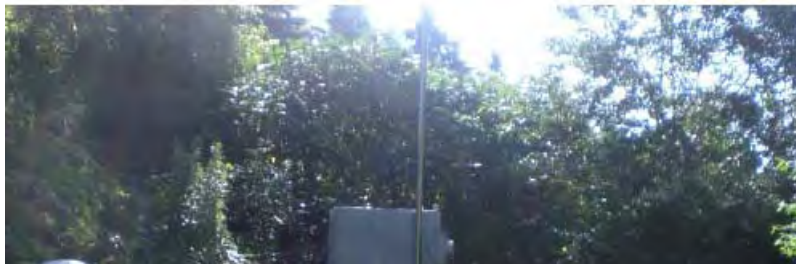
Leighton Way Pump Station to be Replaced
