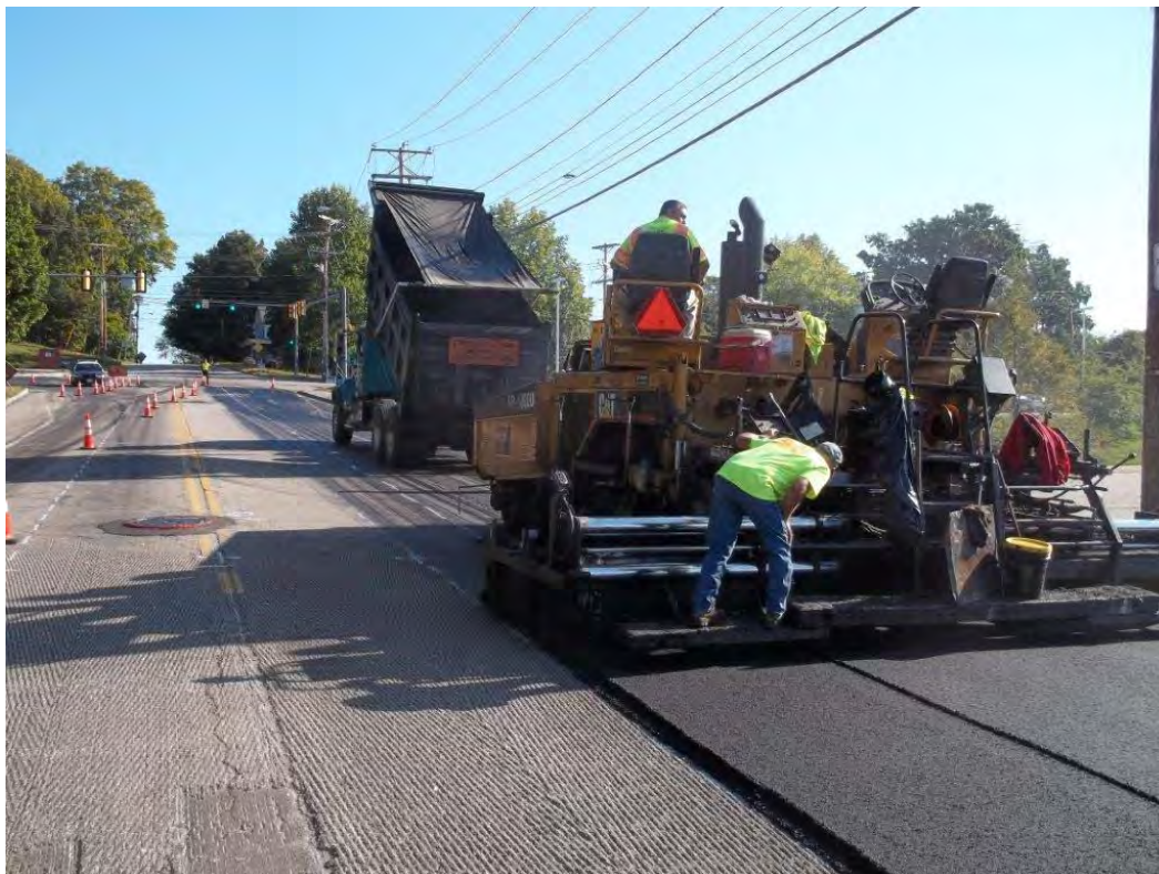
A Roadway Being Paved
