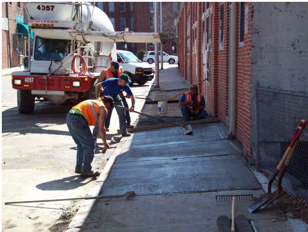
A Sidewalk Being Installed
