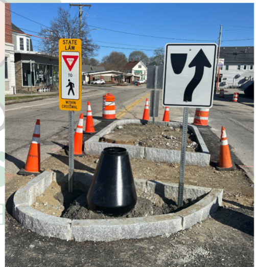
Figure 9: The reconstructed pedestrian refuge island in Central Ave.
