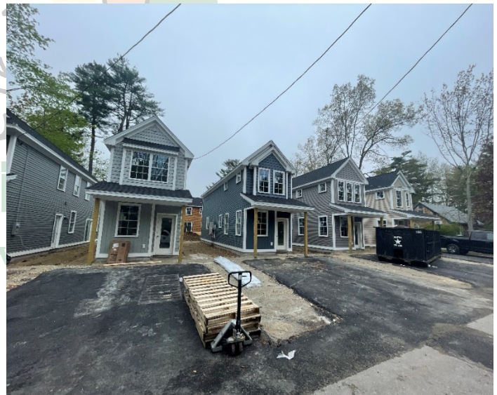
Figure 19: Auburn St. homes under construction.
