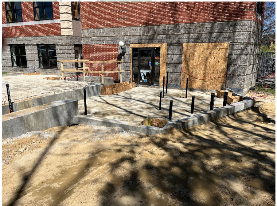
Figure 14: The foundation of the Library expansion area.
