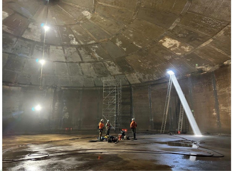
Figure 6: Inside of the 4 million gallon Garrison Hill Tank.
