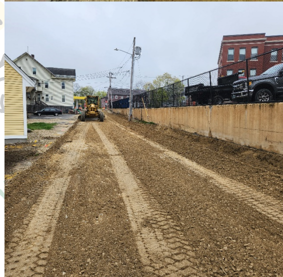
Figure 5: Utility work in Angle Street nearing completion.
