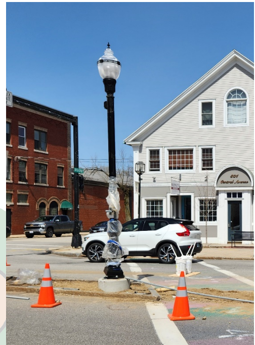
Figure 11: New LED Downtown Lighting is being installed.
