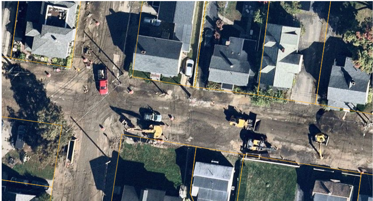
Figure 1: Street reconstruction work on Fifth St.
