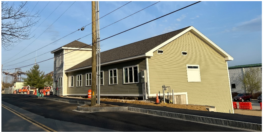
Figure 13: IS Building at Mast Road is almost complete.
