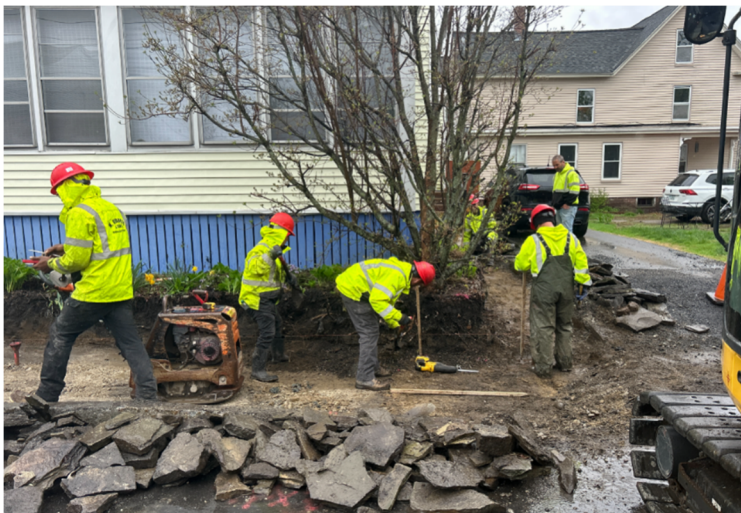
Figure 10: Granese crews rebuilding a retaining wall adjacent to the project area as part of the finish work on Grove Street.
