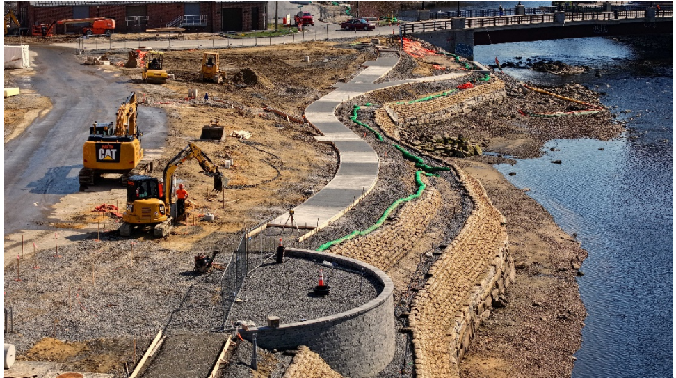
Figure 3: Riverwalk Construction on the Waterfront is moving along.
