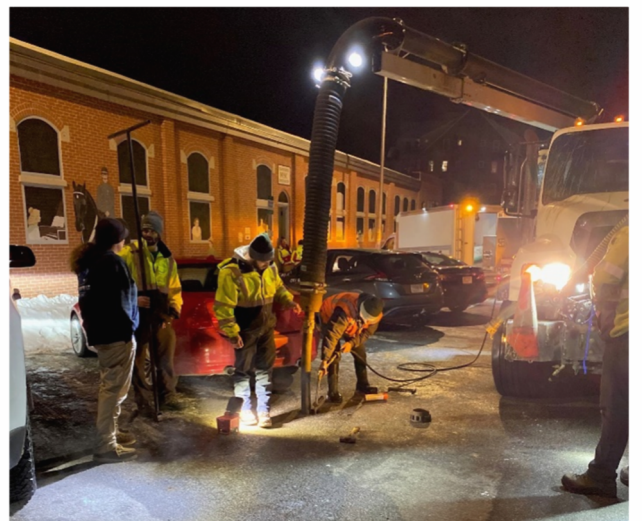
Figure 7: CS crews vacuum out a water shut off in front of the former Earcraft music building during the hunt for a water leak on February 8th.
