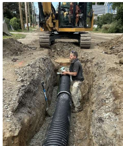
Figure 17: Last section of the 15" drain pipe being installed on Court Street.
