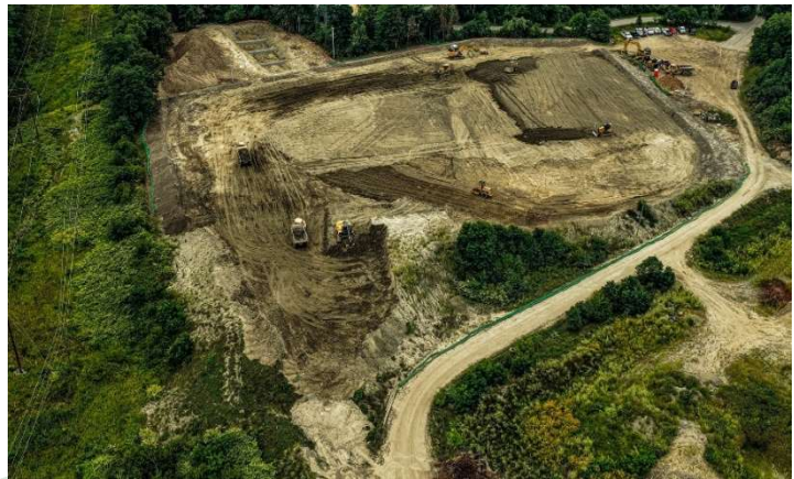
Figure 15: The start of construction.
