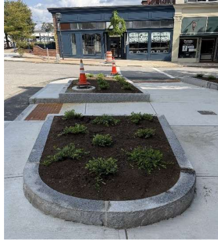
Figure 28: The newly installed bump outs to enhance the pedestrian environment received some greenery last month.
