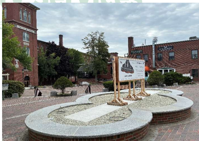
Figure 2: The Cocheco Mill Courtyard is prepared for the memorial installation.
