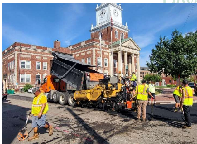
Figure 7: Hale Street paving progress.
