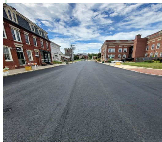
Figure 8: Completed on August 5 th .
