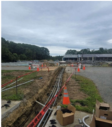
Figure 34: Underground electrical.
