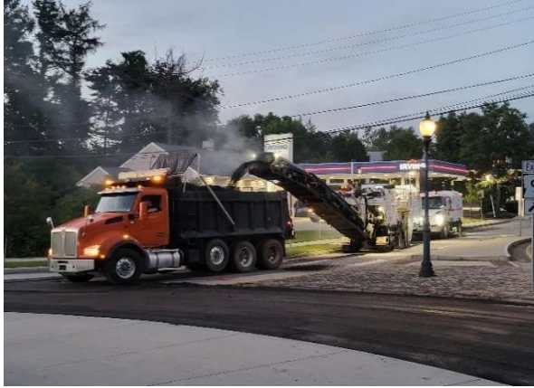
Figure 10: Silver Street milling completed August 23rd overnight.
