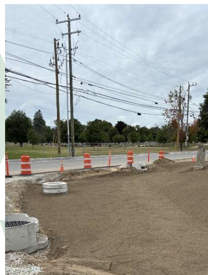
Figure 18: The completed rain garden.
