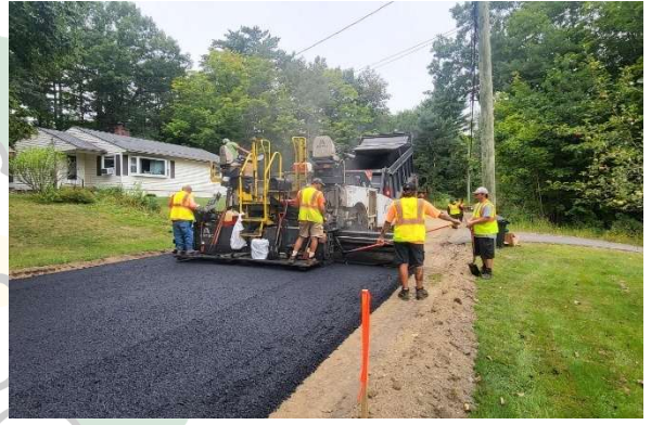
Figure 12: Base paving on Atina. Once completed the Streets Division will grade, loam and seed along the road.
