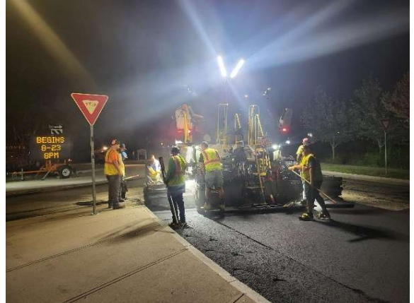
Figure 9: Silver Street Circle paving completed and pavement lines painted on August 31st.
