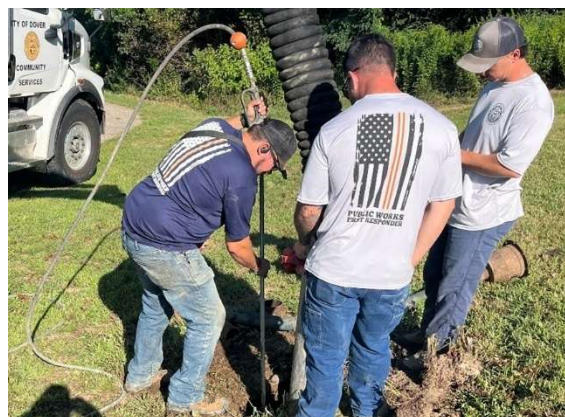
Figure 22: Potholing near an inactive hydrant to assess connection.
