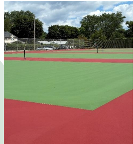
Figure 23: Woodman Park Tennis Courts.
