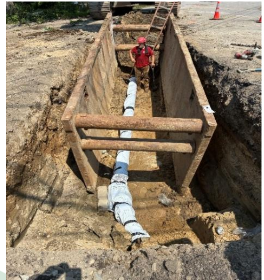
Figure 13: New 8" water main being installed on Back Road
