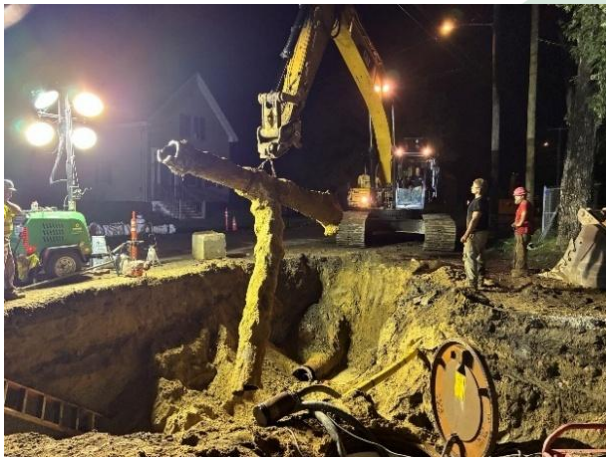
Figure 14: Removal of an old 12" cast iron water main on Court and East Watson. Replaced with a 16" ductile iron main.
