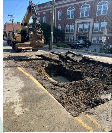
Figure 20: Locust - 8" water main
