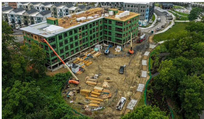
Figure 7: Building F progress.
