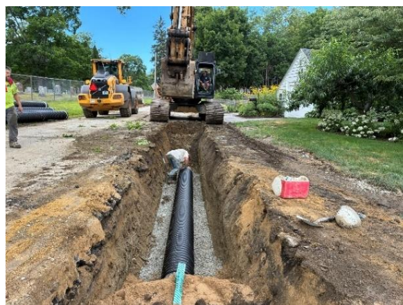
Figure 11: 15" drain pipe being installed to a catch basin on East Watson Drive.
