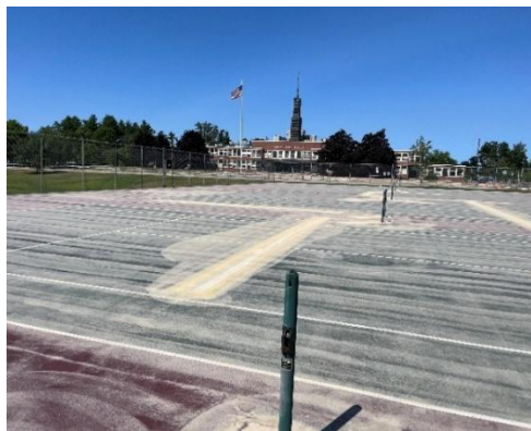
Figure 22: Woodman Park Tennis Courts during maintenance.
