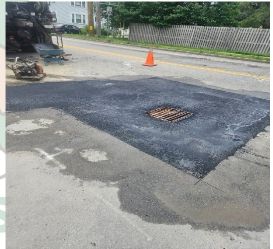
Figure 4: The crew replaced a failed brick catch basin on Oak Street with a concrete structure.
