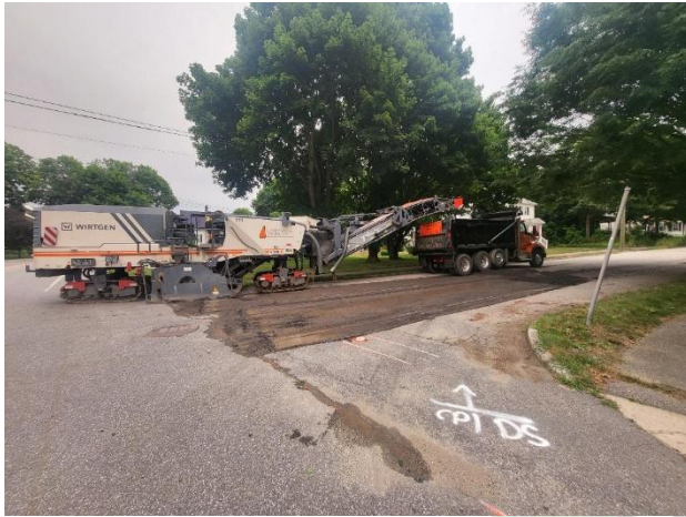
Figure 3: Milling on Towle Ave.
