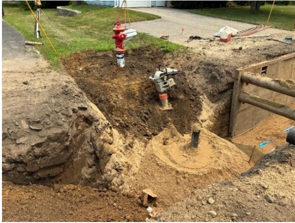
Figure 12: New fire hydrant installed on Court Street at the intersection of East Watson.
