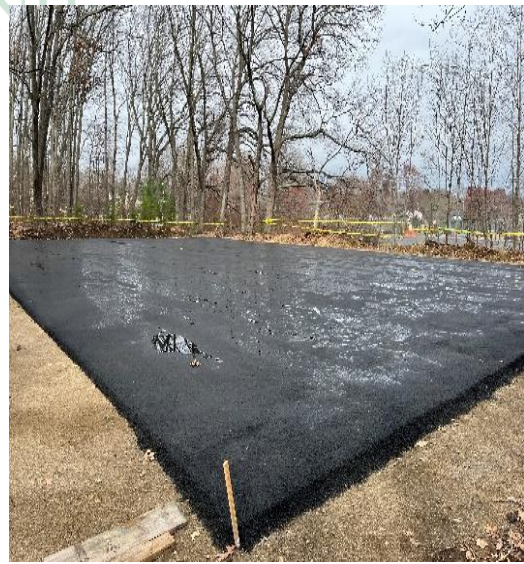
Figure 33: Horne Street Park Basketball courts after pavement.
