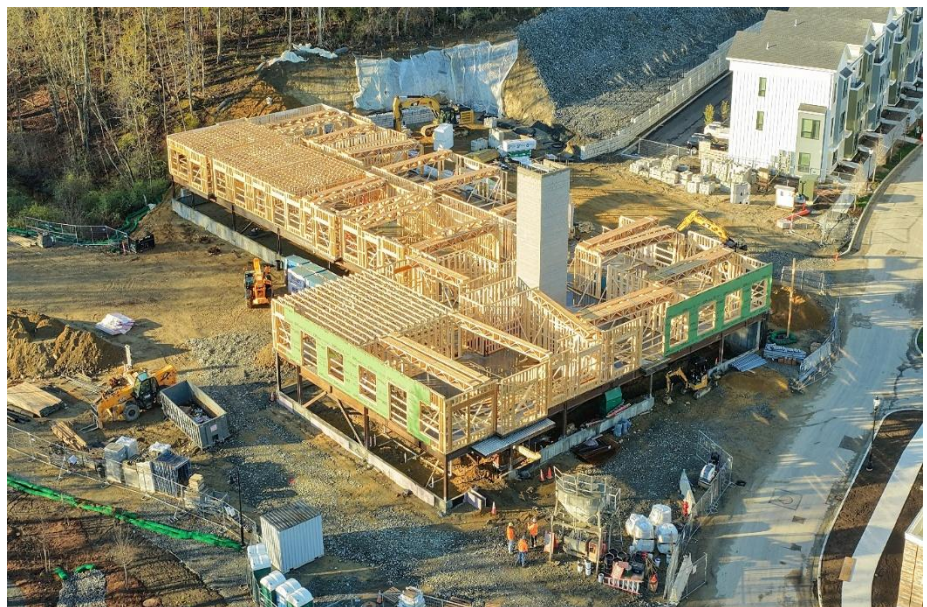
Figure 7: Building F got quite the facelift in the month of April.
