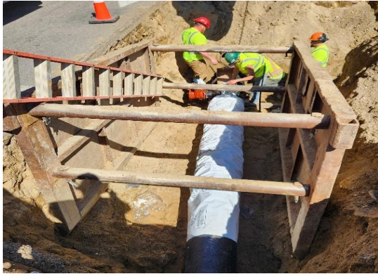
Figure 14: Installation of the new 16" water main on Central Ave.
