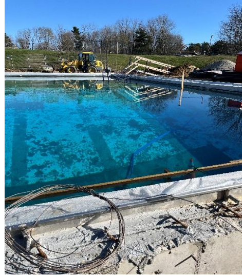
Figure 31: 24 HR Leak Test completed.
