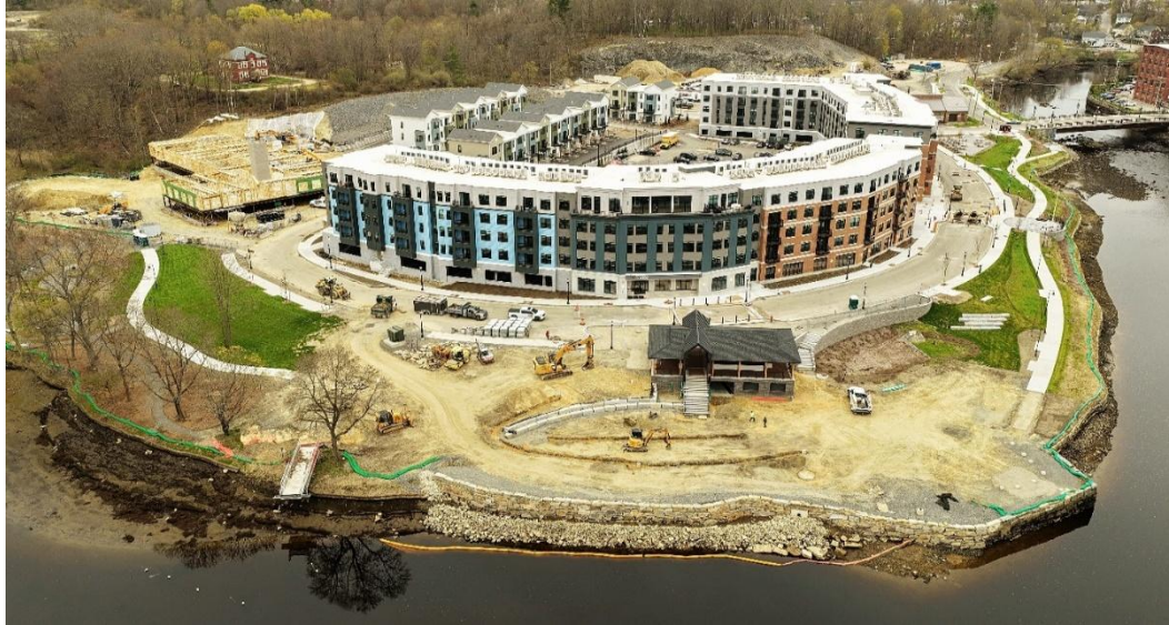
Figure 8: Great progress at the Waterfront in April.
