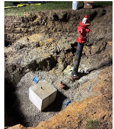
Figure 17: Thrust block and new valve.
