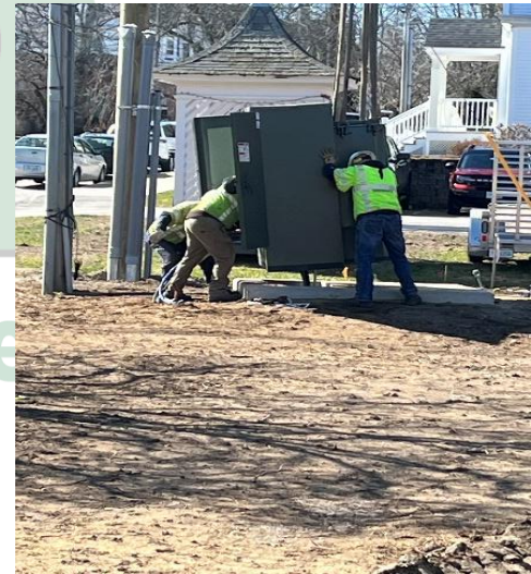
Figure 29: Transformer placement
