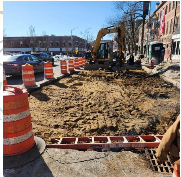
Figure 11: Pavement removal on Central Ave to accommodate a new pedestrian bump-out.
