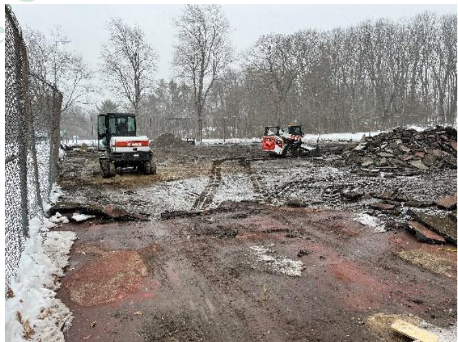
Figure 17: Removal of the tennis courts on Horne Street
