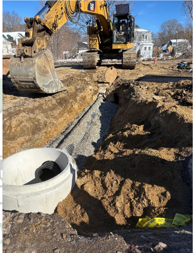
Figure 12: Drainage Infrastructure on Court Street.
