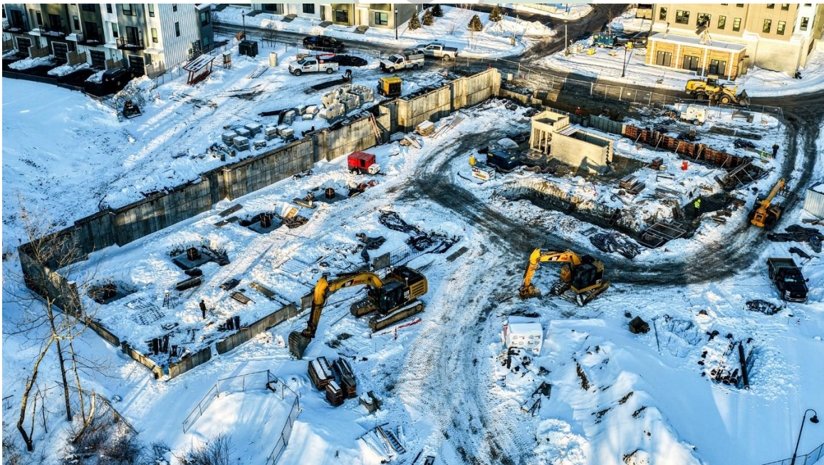
Figure 9: Building F foundation installation.
