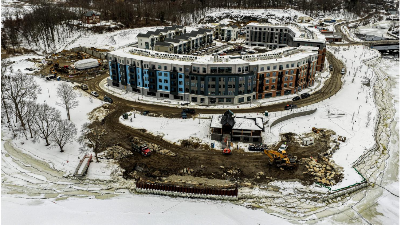
Figure 8: Progress on the Pavilion building and granite toe wall.
