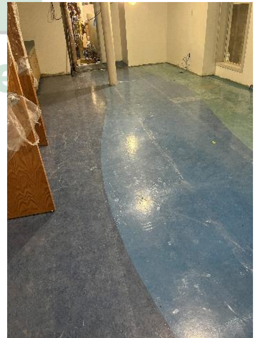
Figure 15: Flooring completed on second and third level
