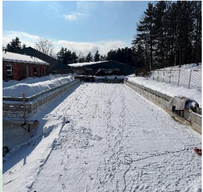
Figure 16: Concrete work to reinforce the Jenny Thompson Pool has been completed
