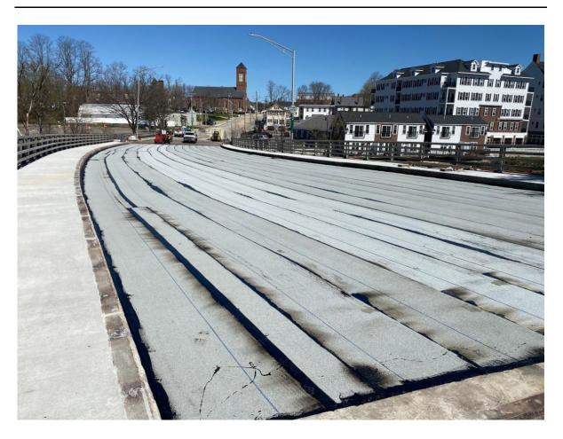
Crews installed the new membrane on the Chestnut Bridge deck. Paving the bridge is set to begin today.
