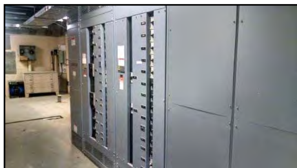
"Transformer room" in Dover High School.
