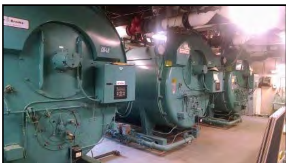
Boiler room at Dover High School.
