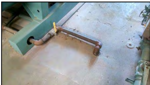
Floor drain adjacent to boiler.
