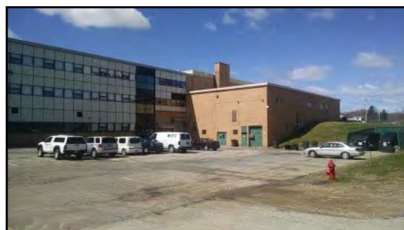
Exterior of Dover High School boiler room.
