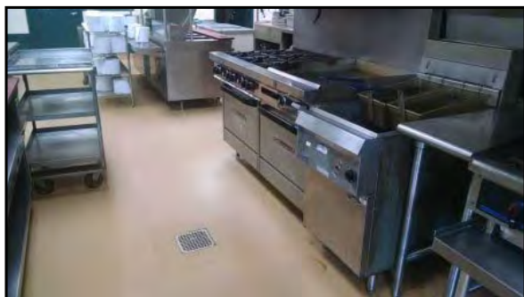
Ovens and floor drain in CTC kitchen.
