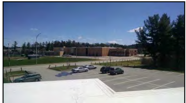
View of the main Dover High School building from the roof of the secondary classroom building.
