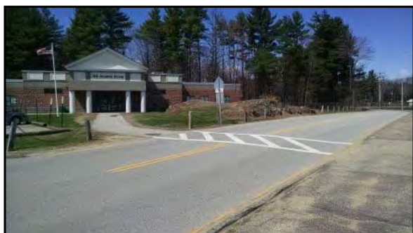
Secondary classroom building.
