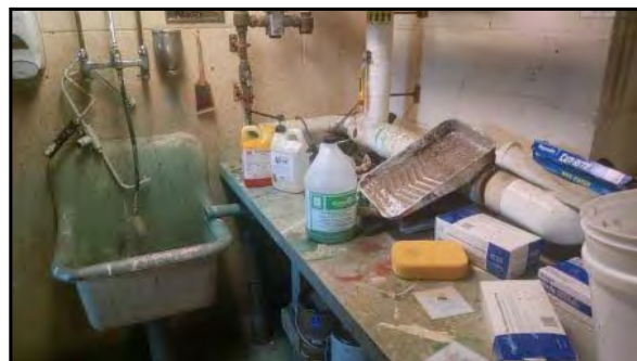
Boiler room at Dover High School.
