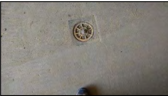
Plugged floor drain in the Maintenance garage.
