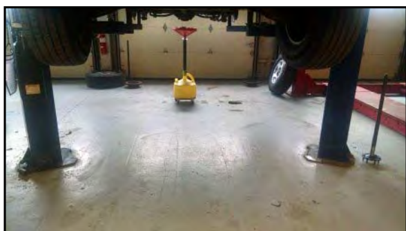
Under hydraulic lift in auto shop.
