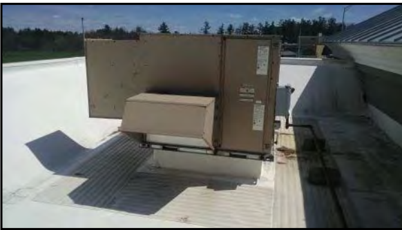
Gas-fired boiler on roof of secondary classroom building.
