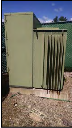
Pad-mounted transformer near athletic field in northern portion of site.
