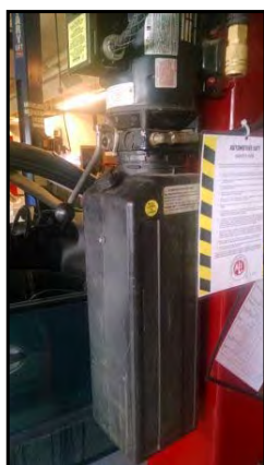
Hydraulic lift in auto shop.
