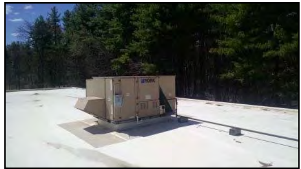
Gas-fired boiler on roof of secondary classroom building.
