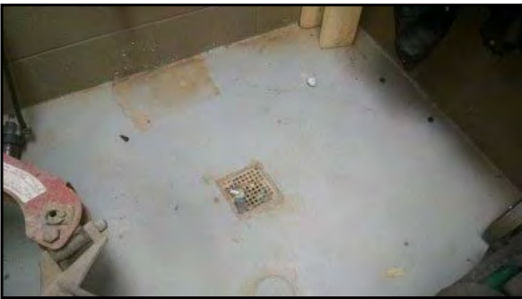
Floor drain in auto body shop.
