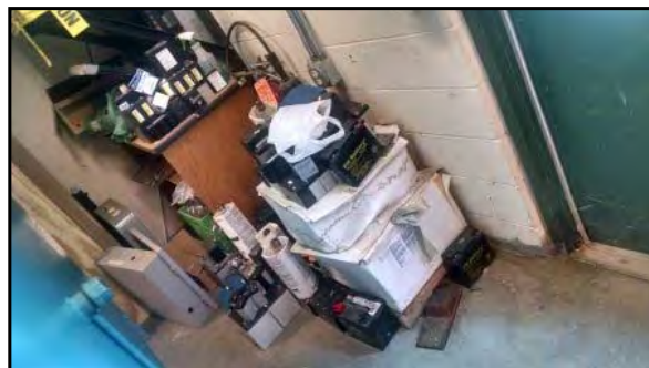
Boiler room at Dover High School.
