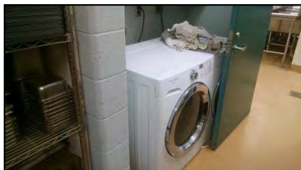
Laundry unit in CTC kitchen.
