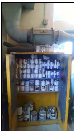
Flammables cabinet in auto body shop.
