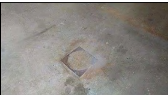
Possible abandoned floor drain in auto body shop.
