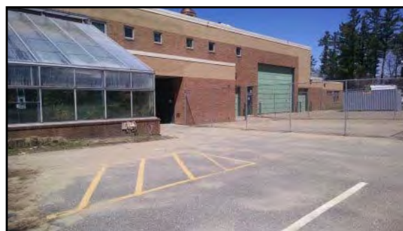
Greenhouse and exterior of the CTC Building.
