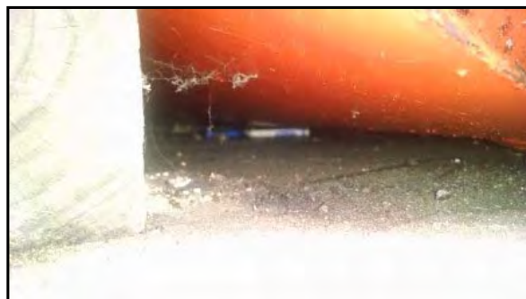
Under the waste oil AST in auto shop in CTC Building.
