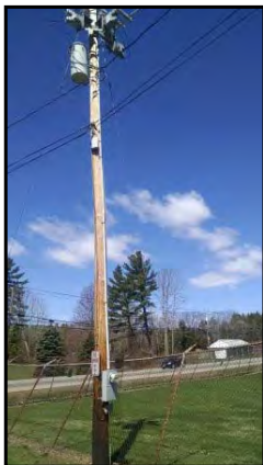
Pole-mounted transformer.
