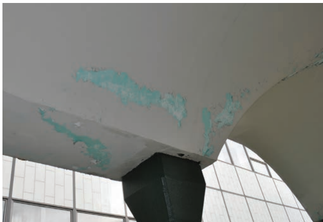
Flaking Plaster at Entrance Canopy
