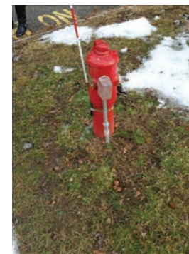
Post indicating valve
