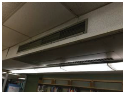
Library Heating & Ventilation Unit
