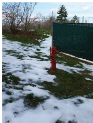
Post Indicating valve
