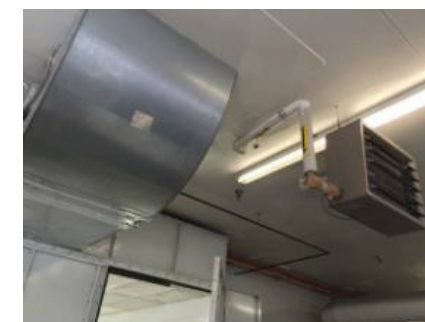
Paint Booth Ductwork and Unit Heater
