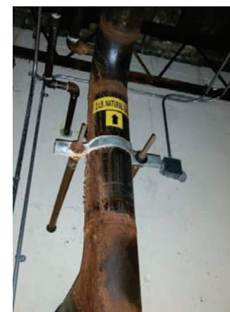
Original building gas piping
