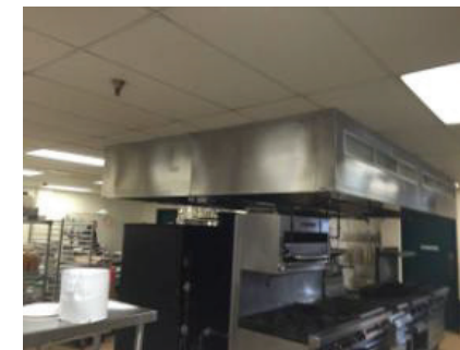
Kitchen Exhaust Hood
