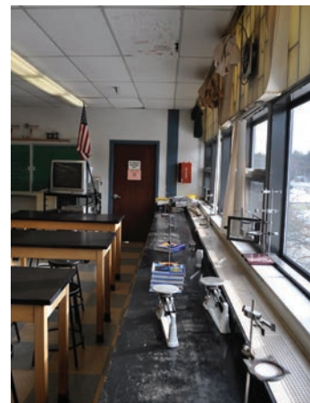
Counter Tops in Disrepair
