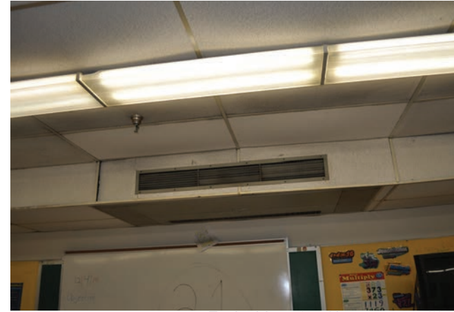
Typical Interior Classroom Ceiling
