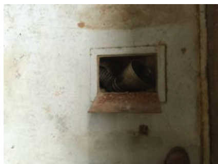
Auto Shop Under Slab Exhaust
