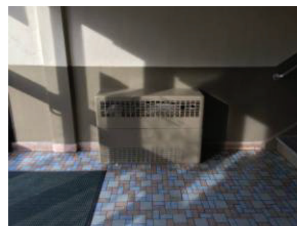
Existing Cabinet Unit Heater
