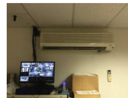
Administration Ductless AC Unit
