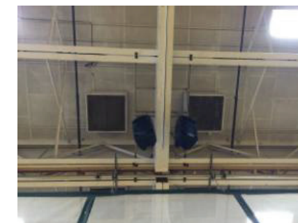
Gym Exhaust Grille
