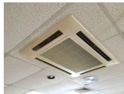
1989 Addition Dining Room Ceiling Ductless AC Unit (typical of 2)
