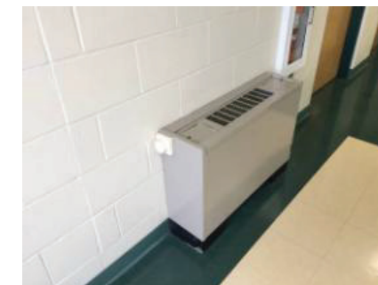
Existing Cabinet Unit Heater – World Arts Wing
