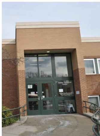
Exterior Wall System 2 - Curtain Wall with Kalwall Infill
