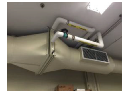
CADD Shop Heating Coil and Ventilation Ductwork
