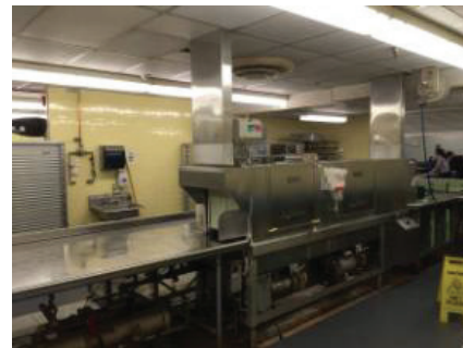
Dishwasher Exhaust Ductwork
