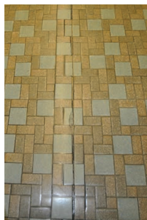
Cracked Tile Floor
