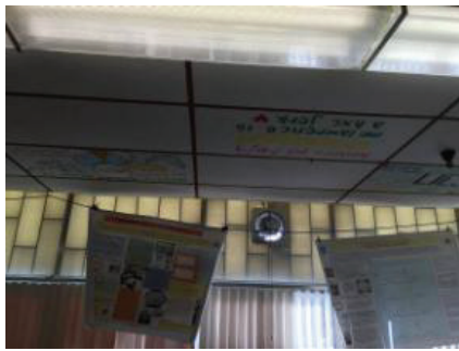
Science Classroom Sidewall Exhaust Fan
