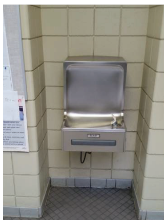
Electric water cooler
