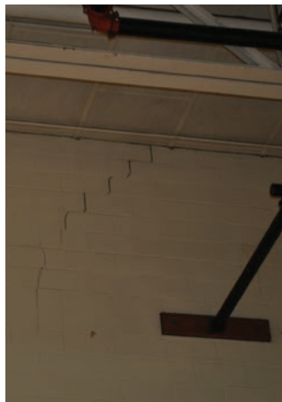
Drinking Fountain, Aged Base Board & Cracking CMU
