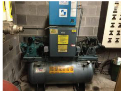
Existing 1989 Addition ATC System Pneumatic Compressor and Control Panel
