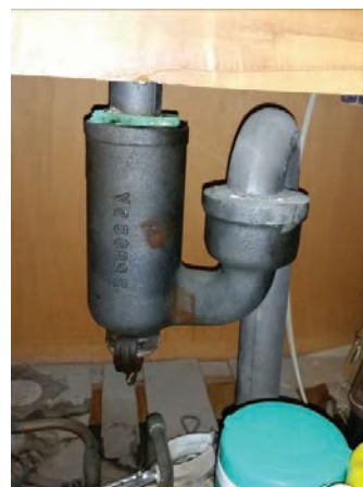
Science waste piping
