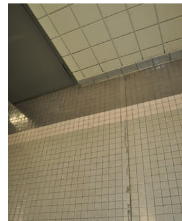
Cracked Tile Floor
