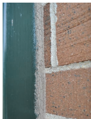
Cracked Sealant
