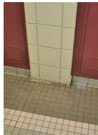
Base in Disrepair
