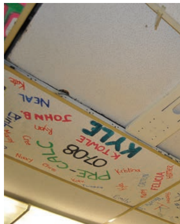
Typical, Painted Ceiling Tiles
