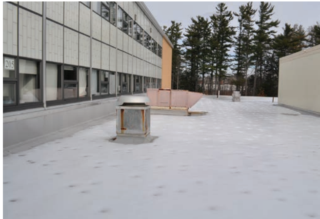
View of Roof with snow cover
