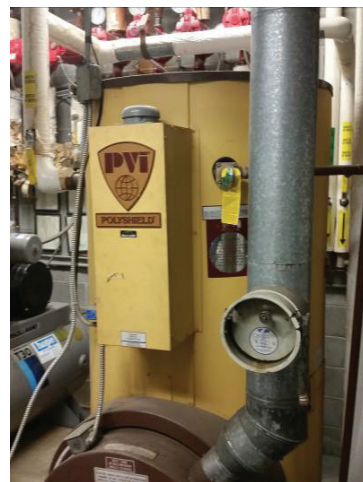
1989 Addition water heater
