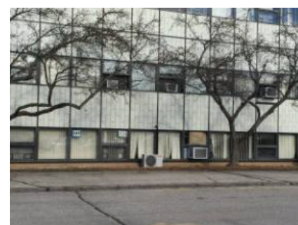
Window AC Units
