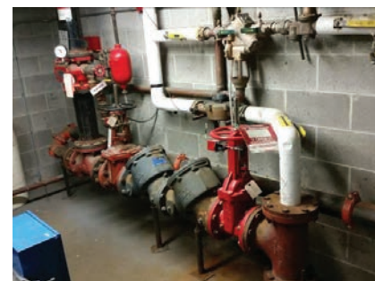
Combined water service - FP riser
