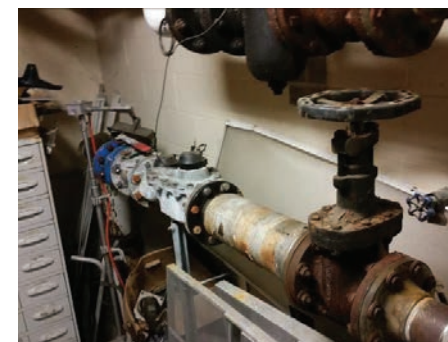
1967 school water service & meter
