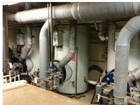
1967 School water heaters
