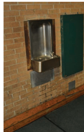
Drinking Fountain, Aged Base Board & Cracking CMU
