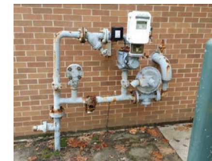
1989 building gas service & meter
