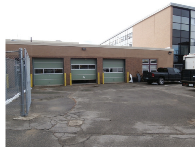
4. Low roof area, north side of 1989 addition, adjacent to three-story 1967 classroom wing.
