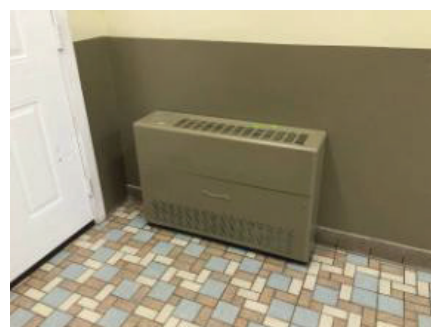
Existing Cabinet Unit Heater
