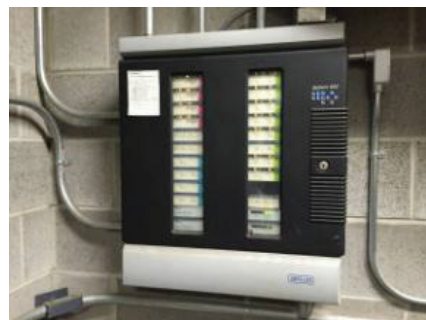
Existing 1989 Addition Building ATC DDC Control Panel
