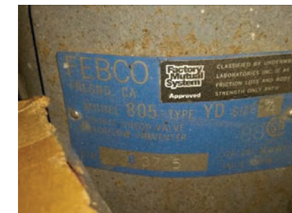
Double check valve assembly
