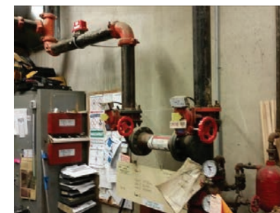
Fire service riser
