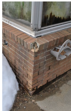
CTC Entrance & Brick in Disrepair
