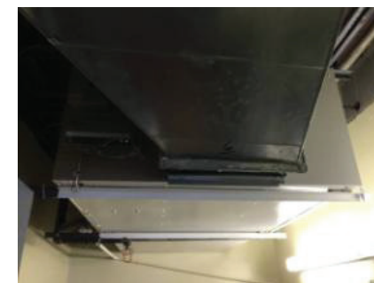
Administration Air Handling Unit
