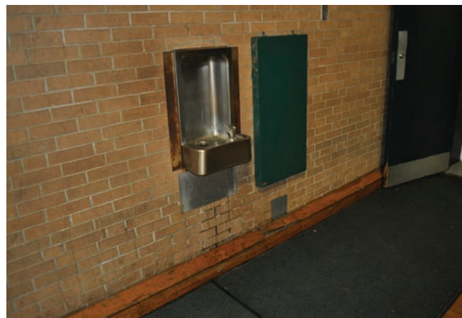
Inaccessible Water Fountain
