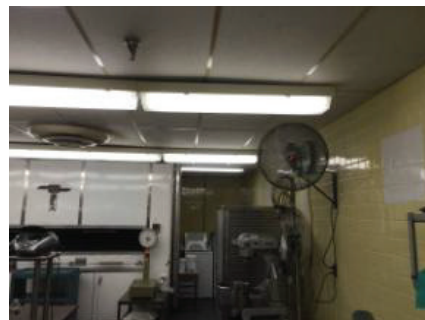
Supply Diffusers (left) and Prop Fan (right)
