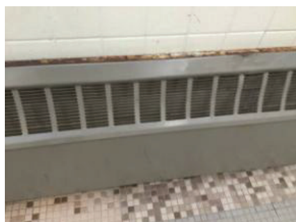
Locker Room Fin tube Radiation
