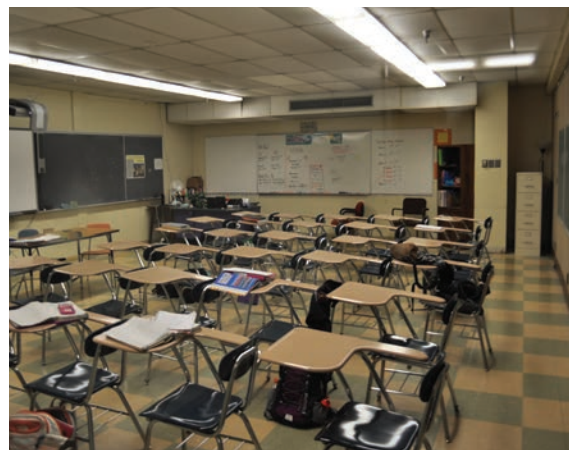
Typical Classroom - Asbestos Tile Floor
