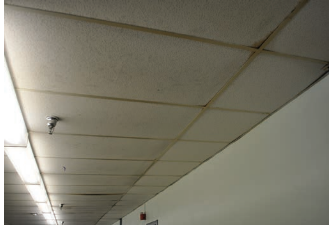
Typical Corridor Ceiling in Disrepair
