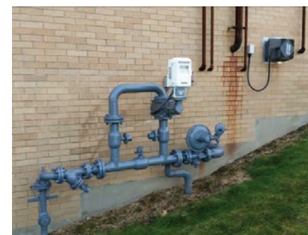
Original building gas service & meter
