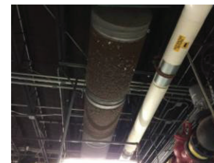
Combustion Air Perforated Supply Diffuser
