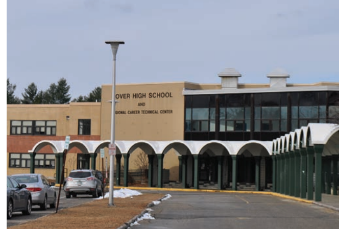
View of Entrance Canopy
