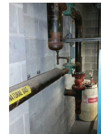
1989 building gas piping
