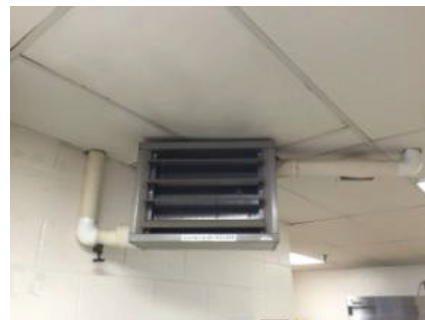
Kitchen – Unit Heater
