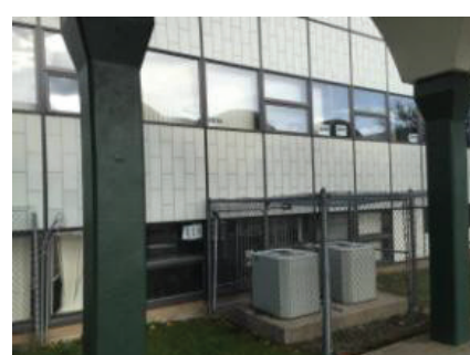
Grade Mounted Air Cooled Condensing Units
