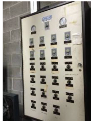
Existing 1989 Addition ATC System Pneumatic Compressor and Control Panel
