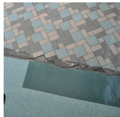
Missing Expansion Joint at 2002 Addition
