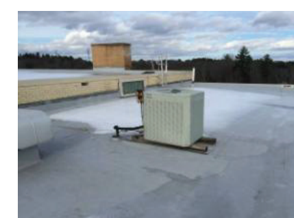
Roof ACC Unit
