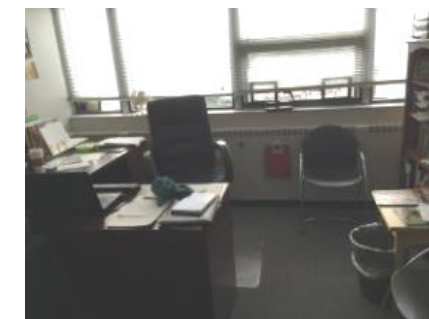
Administration Office – Fin tube Radiation Heating
