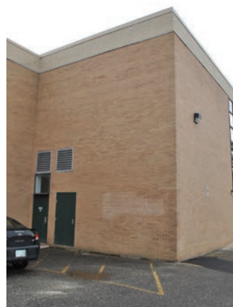
Visible Efflorescence
