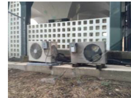
Ductless AC Unit ACC Units
