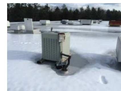
Roof ACC Unit
