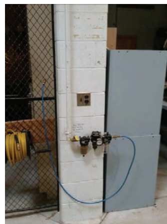
Typical air outlet station
