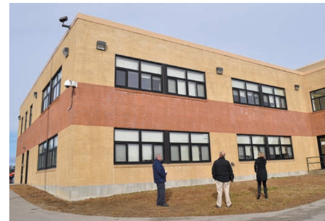
2002 Addition with Visible Efflorescence
