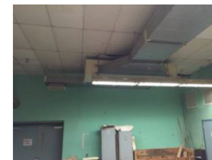
Wood Shop Unit Ventilator
