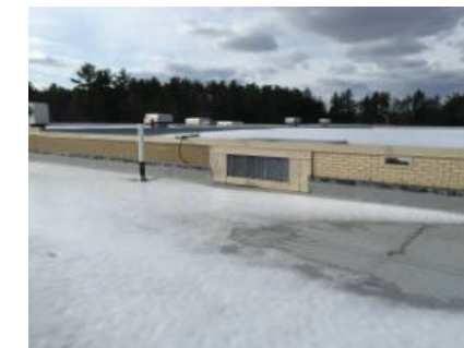
Unit Ventilator Intake Louver
