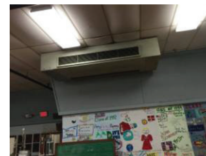
Music Classroom – Unit Ventilator
