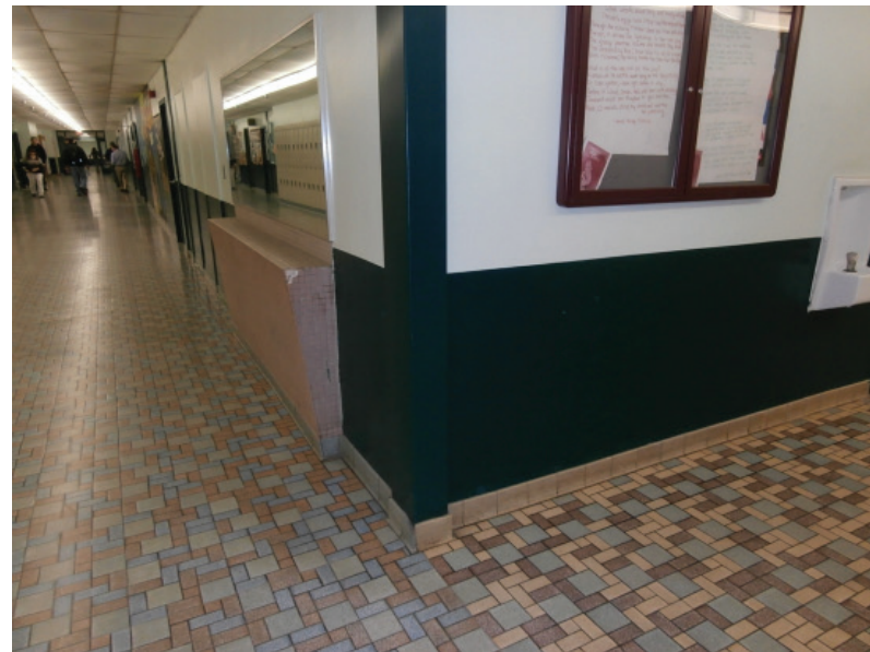
9. 1967 Classroom Wing – corner column at corridor intersection.
