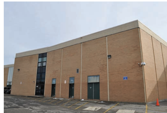
Exterior Wall System 1 - Brick Veneer
