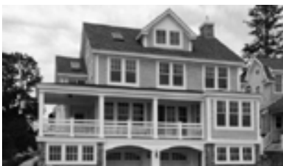
Varied rooflines and dormer adds visual interest.
