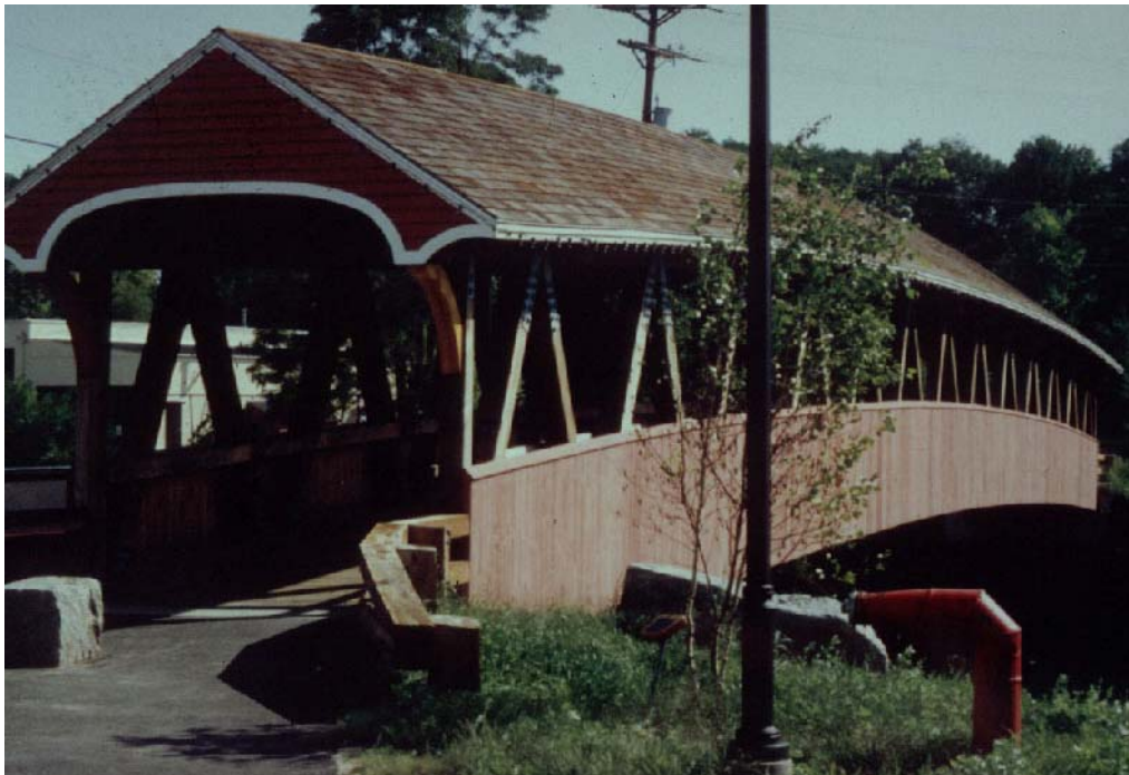
Cochecho River Pedestrian Bridge Linking Waterfront Area and Downtown Dover
