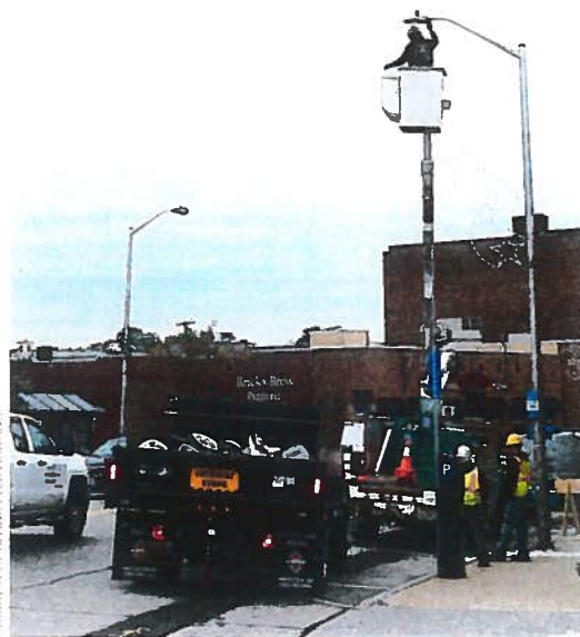
Installation of Affinity LED Lighting in Dover.
