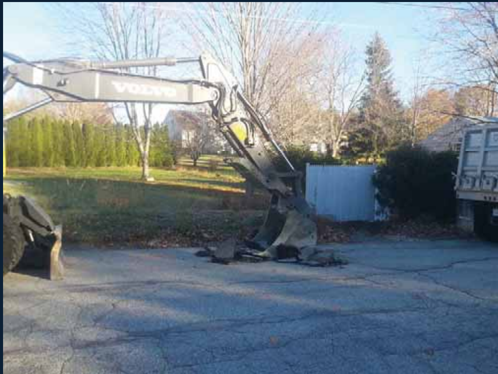
Existing Asphalt Removal
