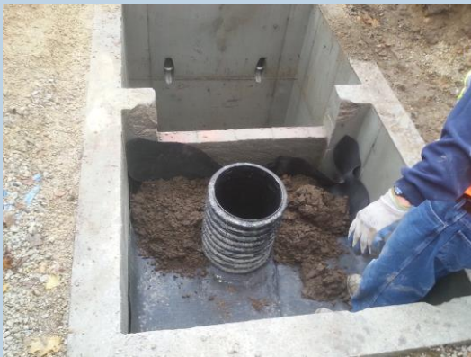
Photograph 3: Roosevelt Avenue filtering catch basin 1.
