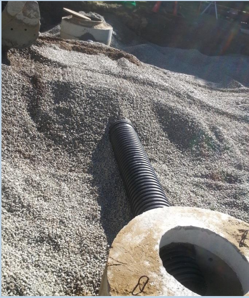
Photograph 4: Grove Street subsurface gravel filter.
