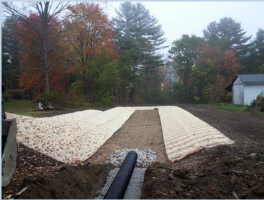
Photograph 2: Bioretention system at lower Horne Street
