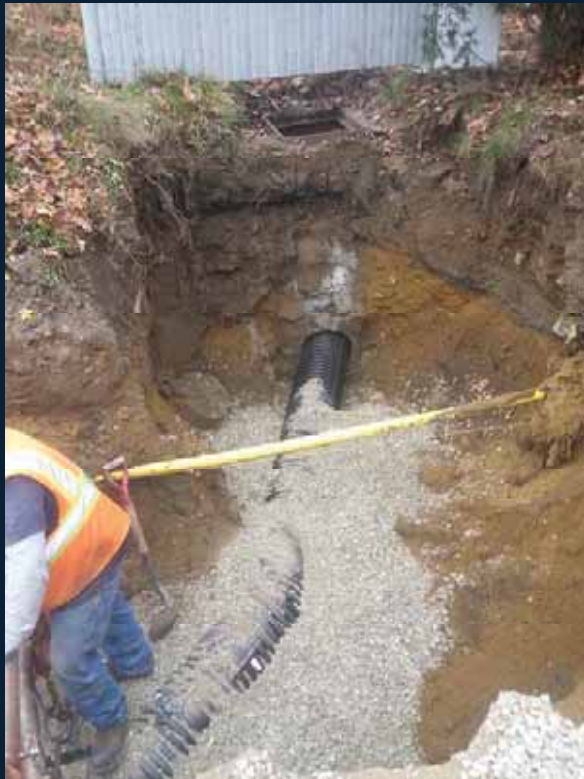
Outlet pipe installation
