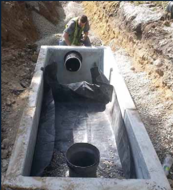
Media Box Filter with geotextile and pipe installation
