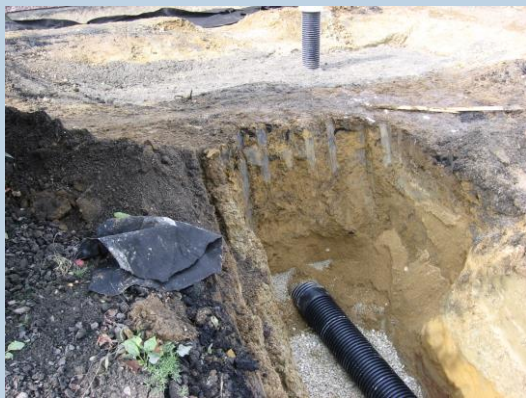
Photograph 5: Hillcrest Avenue infiltration trench.
