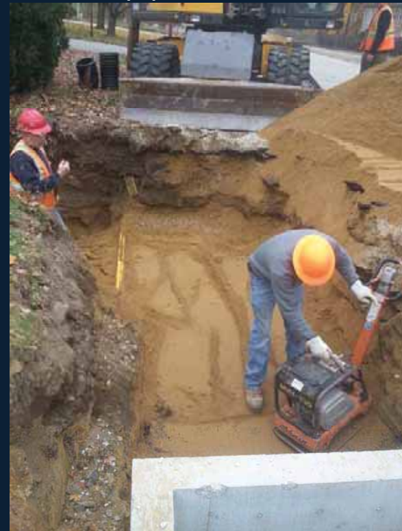
Backfill and compact over outlet pipe installation
