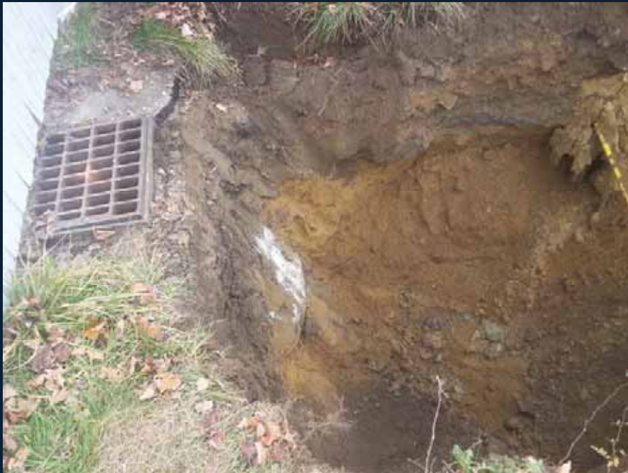
Additional excavation to install outlet pipe
