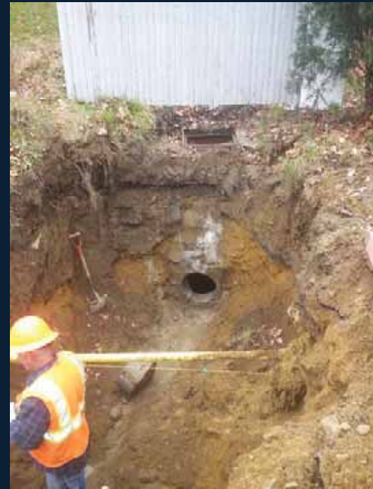
Core hole in existing structure for outlet pipe installation
