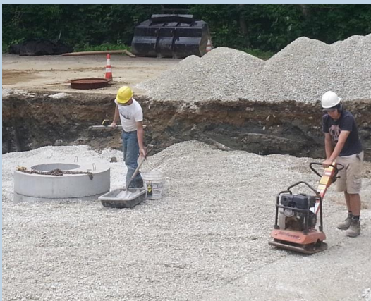
Photograph 7: Kettlebell Subsurface Gravel Filter
