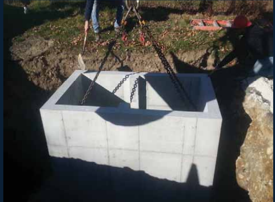
Placement of Media Box Filter
