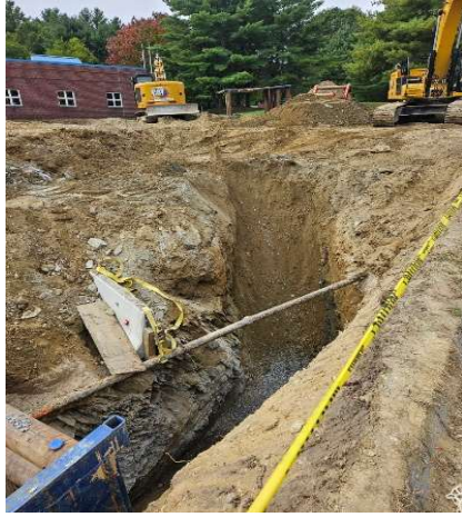
Figure 38: Trenching and ledge removal process.
