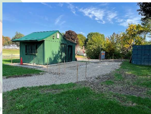
Figure 35: ADA parking improvements.
