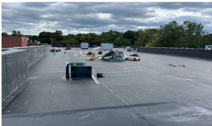
Figure 33: Structural support work on the roof at McConnell Center.
