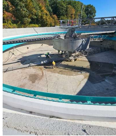
Figure 37: New grout applied to the clarifier floor.
