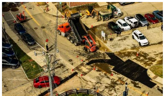
Figure 10: Temporary Patchwork.
