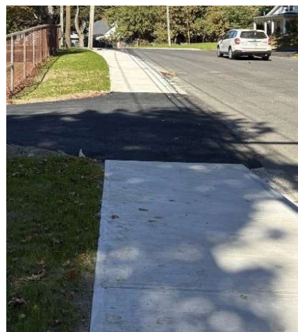
Figure 16: Sidewalk installation on Court Street.
