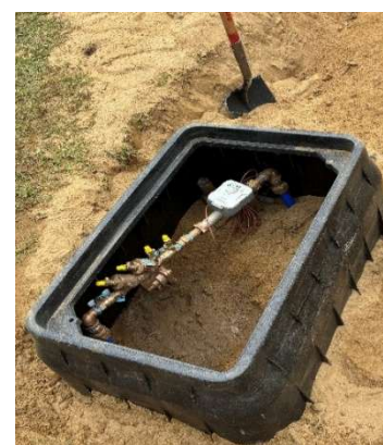
Figure 26: Hot Box installation for the new meter.
