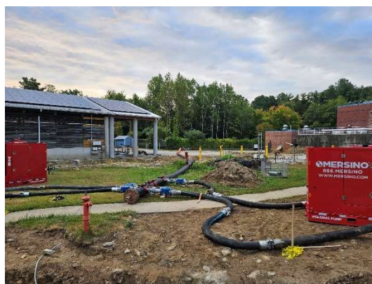
Figure 36: Bypass pumping.
