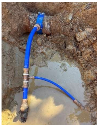
Figure 27: Potholing for the WSLI project.
