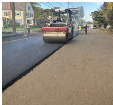
Figure 18: Court Street base paving.
