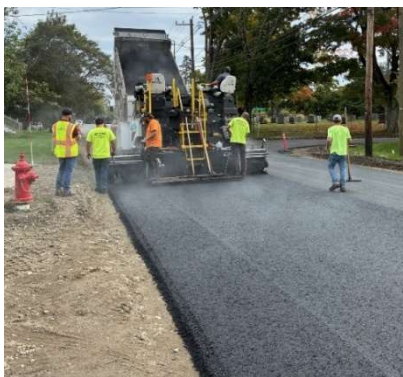
Figure 19: Court Street base paving.
