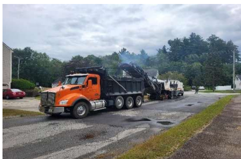
Figure 6: Milling on Pondview Drive.
