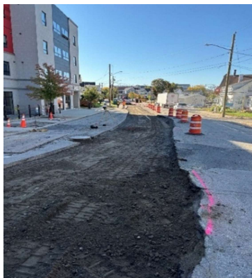
Figure 21: Water Main installation progress.
