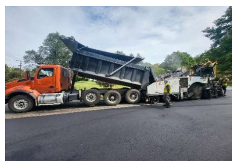
Figure 7: Paving of Chandler Way.
