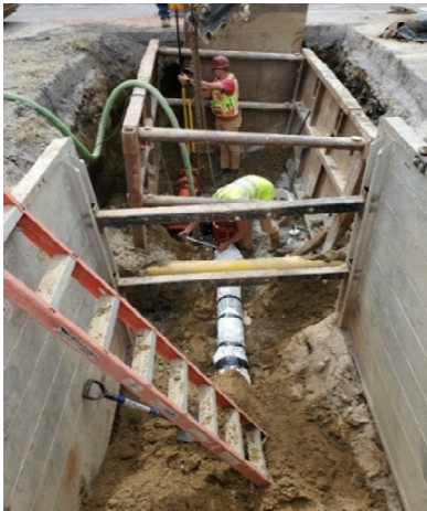
Figure 14: Water main with protective wrapping.
