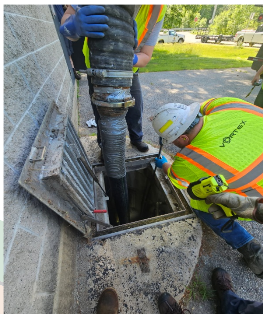
Figure 40: Crews performing routine maintenance.
