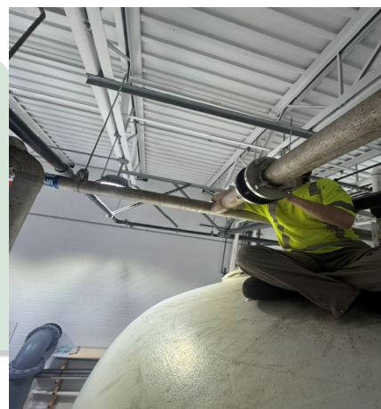
Figure 23: Lowell WTP Filter 2 check valve installation and final repairs completed.
