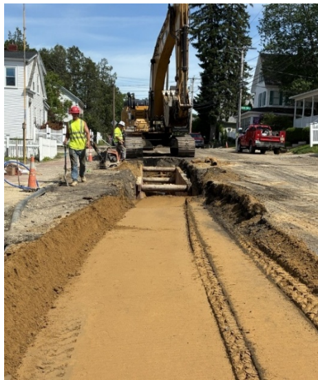
Figure 9: Grading and compaction of a typical water trench.
