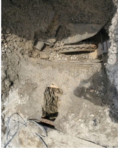
Figure 12: Water main underneath electrical duct bank.
