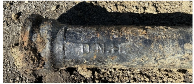
Figure 8: A rarity for this time period for City's and Town to have cast iron water pipes. The manufacturers made sure it was properly stamped for a specific destination for installation.
