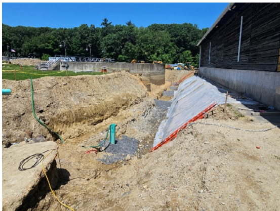
Figure 38: Site work progress.
