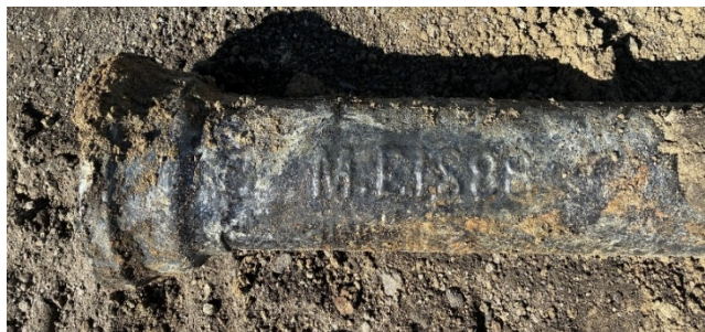
Figure 7: The above and below images show the old cast iron water main that was removed from Court Street, dated 1888.
