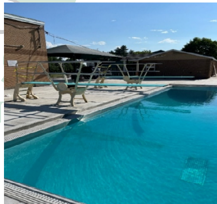
Figure 33: Newly installed diving boards.
