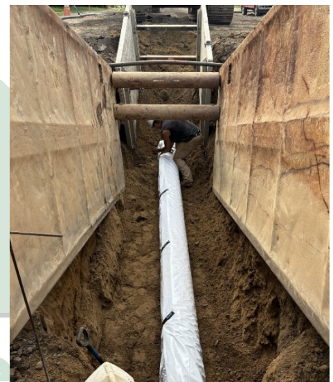
Figure 10: Installation of a new water pipe in a trench box (for safety purposes) with a wrap for external corrosion control.
