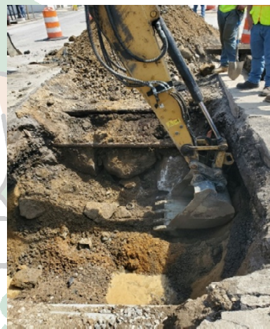
Figure 15: Site work for pipe repairs.
