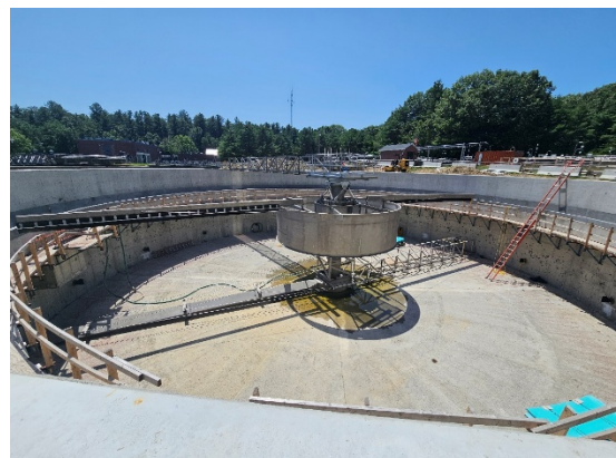
Figure 39: In place and almost ready for action.
