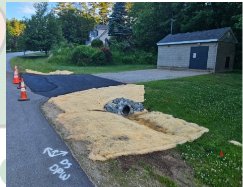
Figure 37: Site prep, install and finishing touches of the new culvert.
