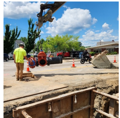
Figure 11: Valve assembly for the new water main installation.
