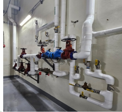
Figure 36: Completion of the jacket process.
