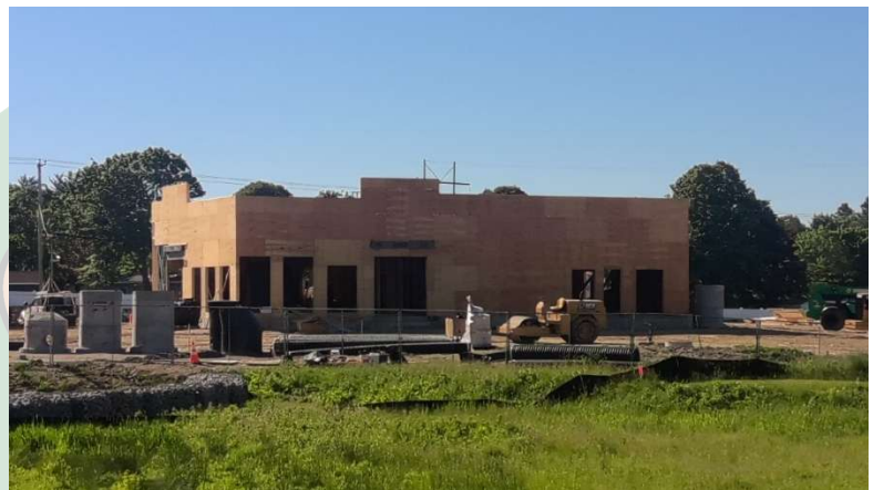
Figure 17: McDonalds on Grapevine Drive construction progress
