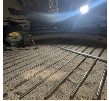
Figure 26: New media in place.
