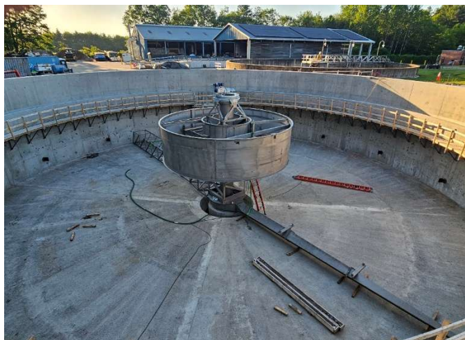
Figure 43: Install of Clarifier Mechanism.
