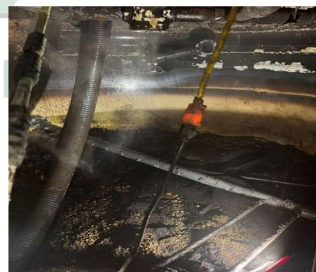
Figure 24: Repairs to the air filter area.
