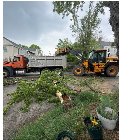
Figure 34: Streets Division and Facilities, Grounds and Cemeteries performing tree
