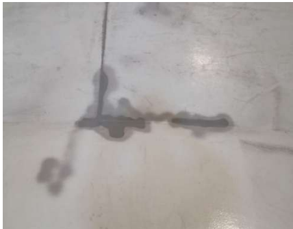
Figure 29: Before the walls were repaired.
