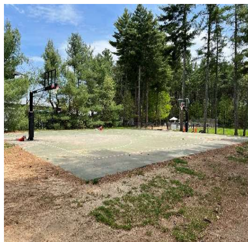
Figure 39: New Basketball hoops installed at Long Hill Park.
