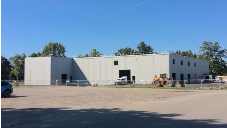
Figure 16: 34 Industrial Park site work progress
