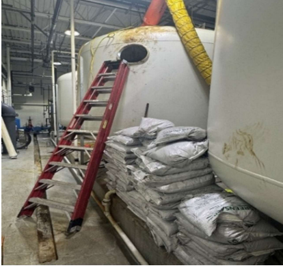
Figure 27: Staff hauled bags to fill the filter.
