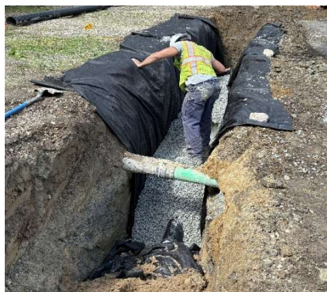
Figure 12: New underdrain pipe with fiber mesh wrap and crushed stone for support.
