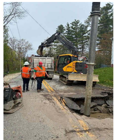
Figure 18: Garrison Road water main repair.
