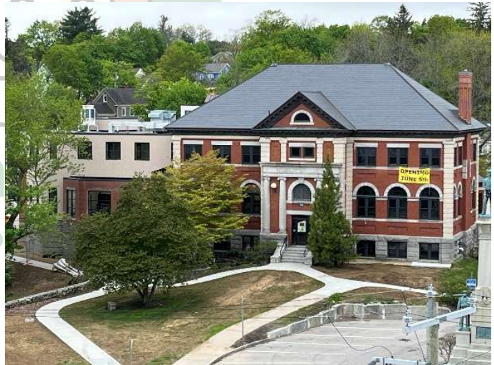
Figure 36: Library as we progress into June.
