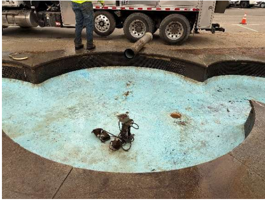
Figure 19: Crews using the vector truck to remove soil.
