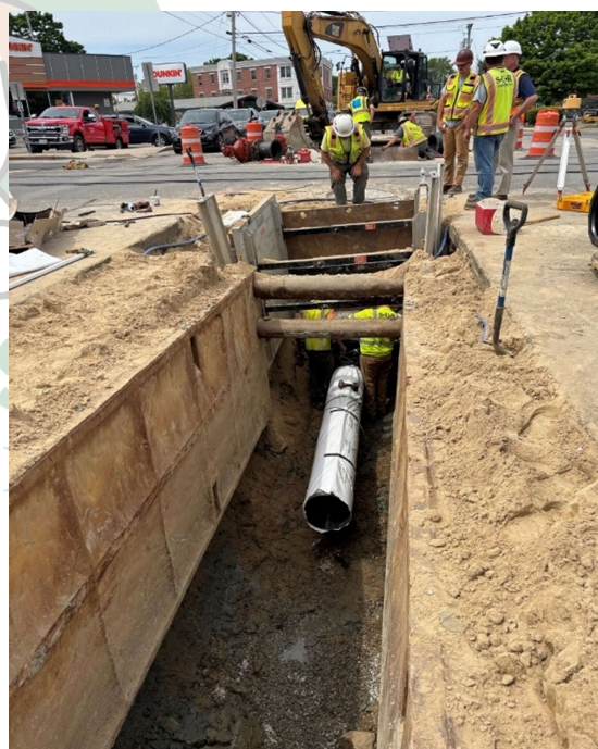
Figure 14: Water main installation.
