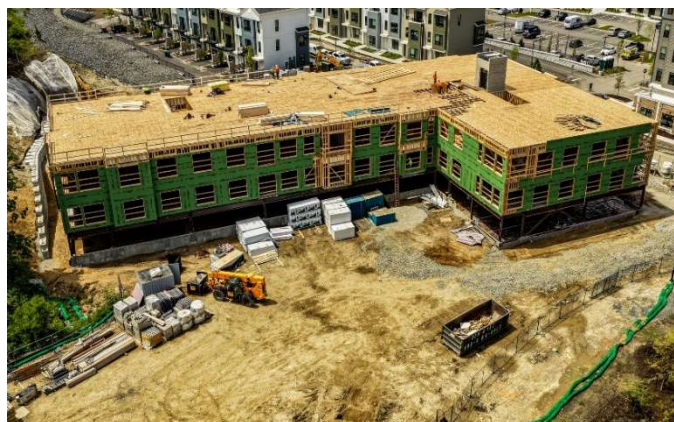
Figure 9: Building F is coming to life.
