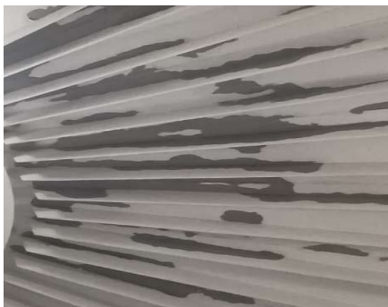
Figure 30: Before the roof repairs.
