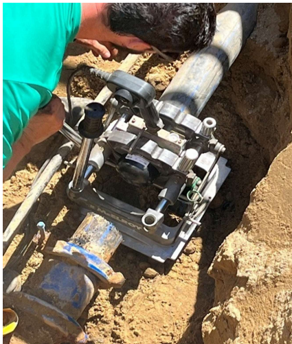
Figure 22: Utilities completing the install.
