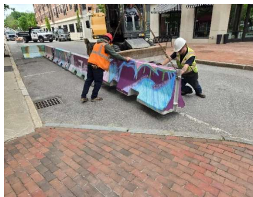
Figure 3: The Crew working out front of the Nook.
