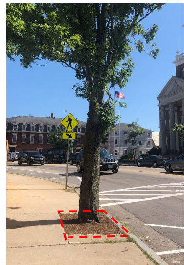
Figure 5. Tree pit, also referred to as a tree box or tree well
