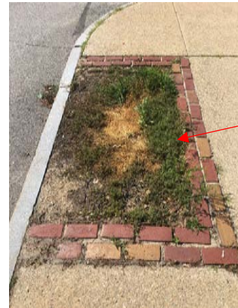
Figure 3. Empty tree pit
