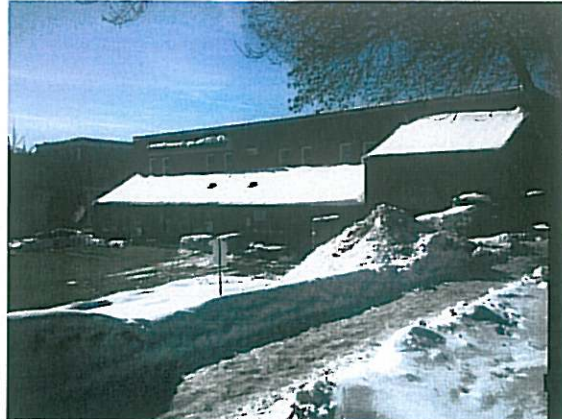
South End of Property Looking Southwest to Aubuchon Hardware (~15 elevation change)
