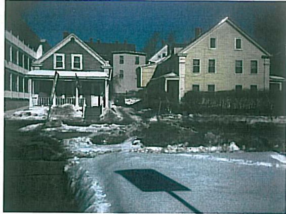
Northwest Entrance of Property Looking North Across 1 st Street
