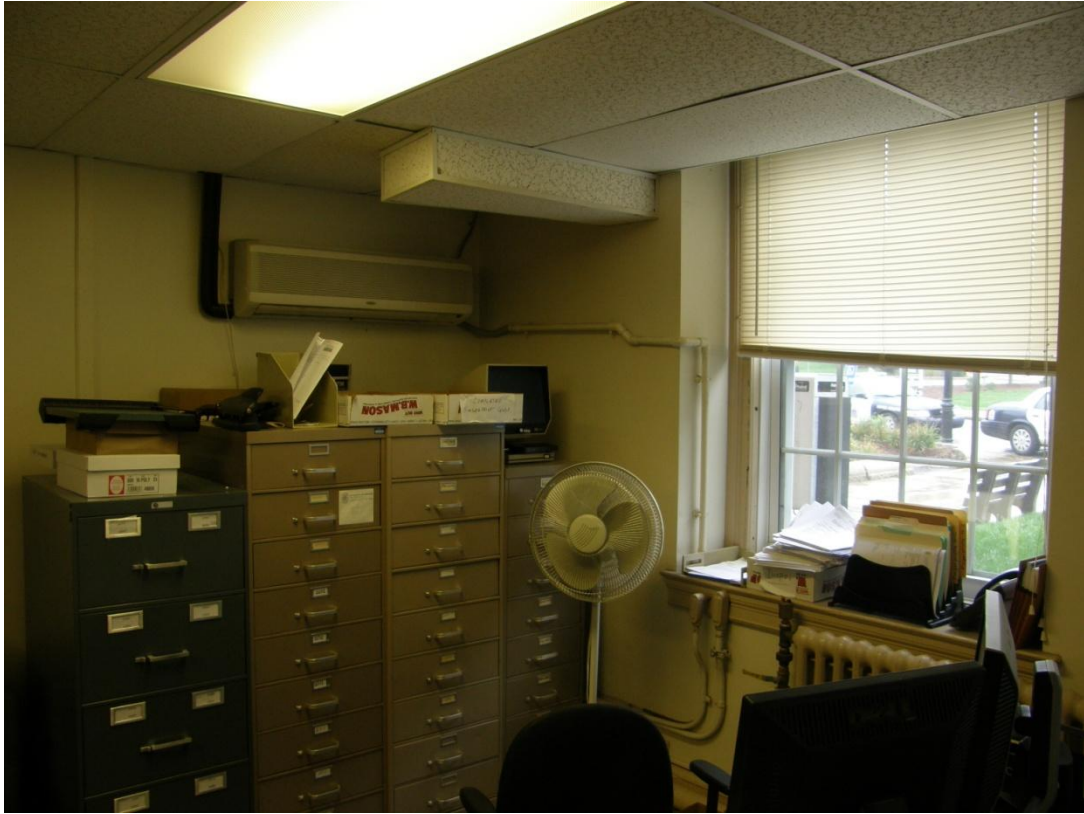
Interior view of unfortified window in Records Bureau office
