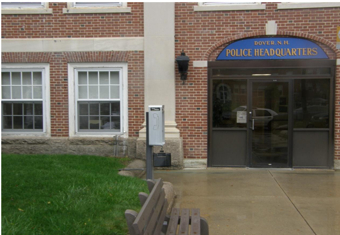
Exterior view of unfortified windows in Records Bureau office
