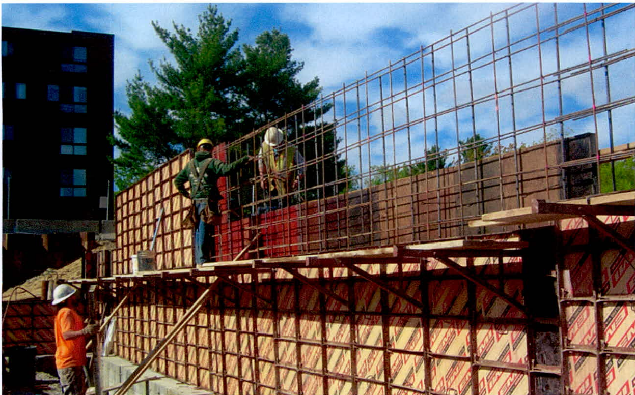
Installation of poured concrete foundation wall of garage structure – June 2015.
