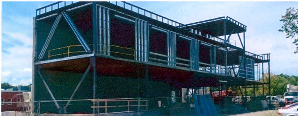
North façade of police building – August 2015.
