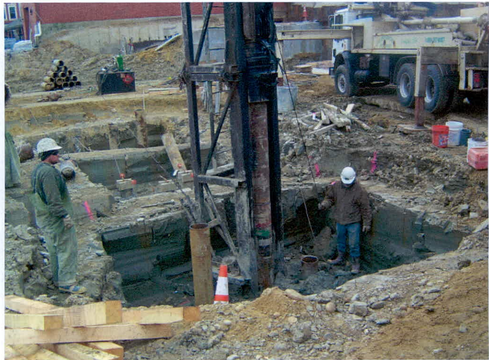
Installation of Building Support Piles – April 2015.
