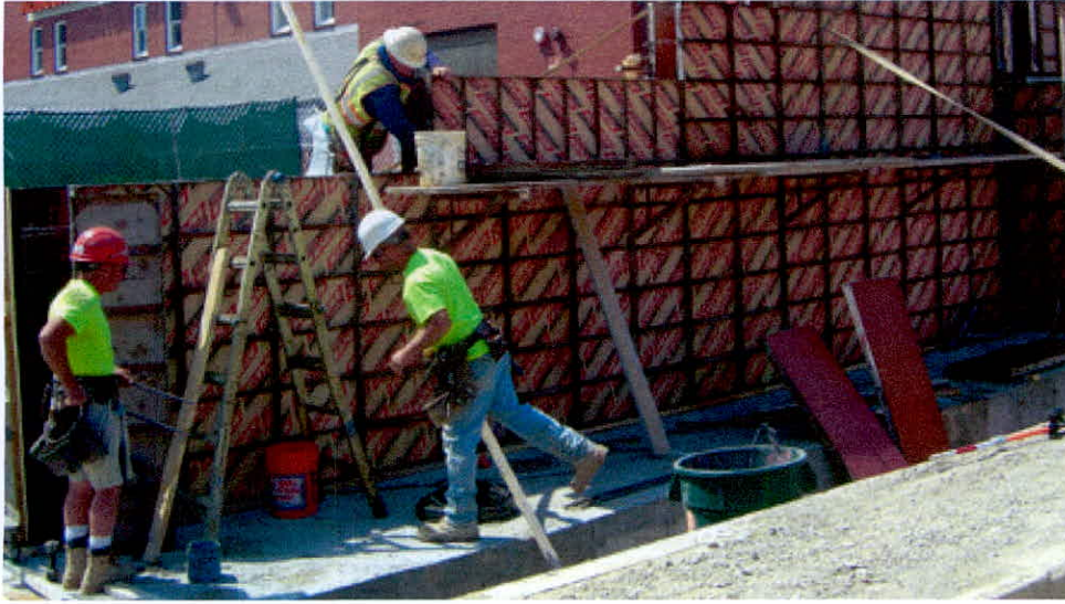
Construction of South foundation wall of parking garage – May 2015.
