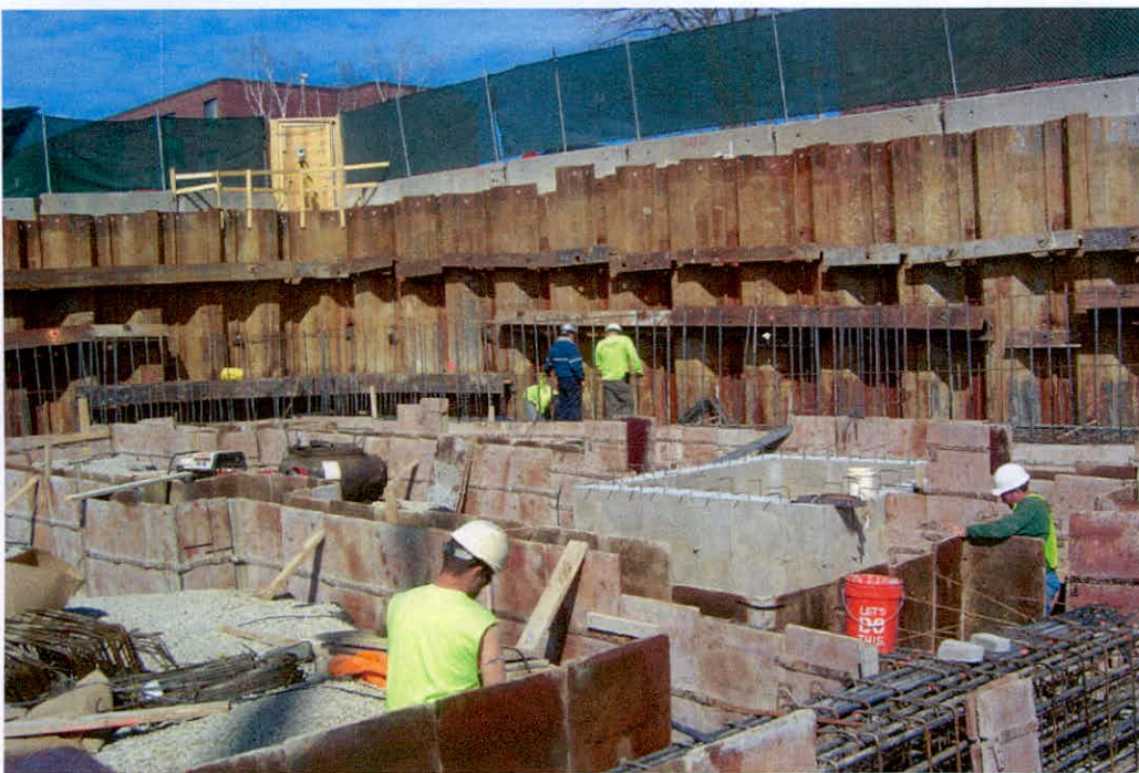
Installation of footing grade beams for police building – May 2015.
