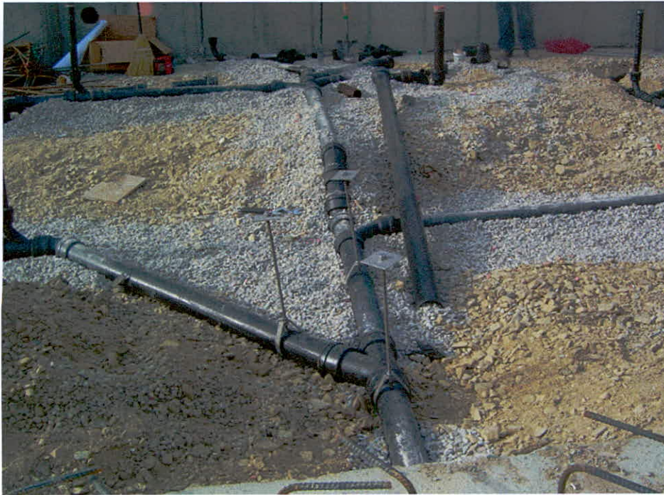
Under slab plumbing in police facility prior to concrete placement – June 2015.
