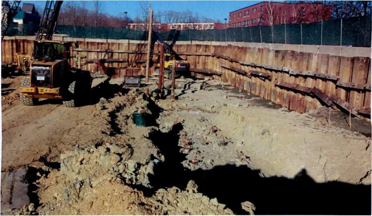
Installation of building support piles in Northwest corner of site – March 2015.
