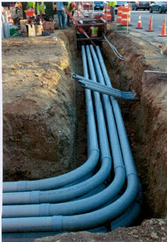
Crews move underground utilities – October 2014.
