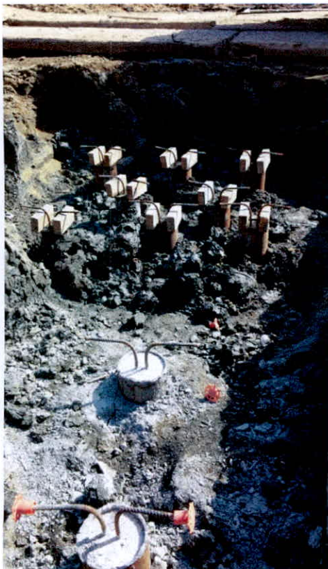
Installed Building Support Piles.
