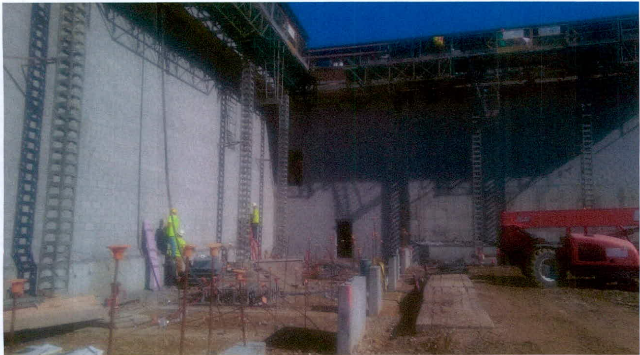
Construction of block fire wall between police and garage structures – August 2015.
