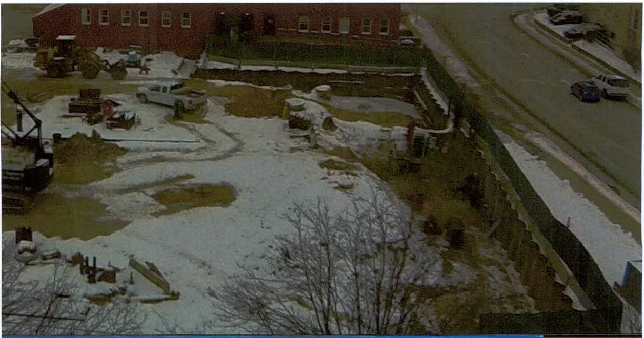
Excavation begins along the West side of the site – December 2014.
