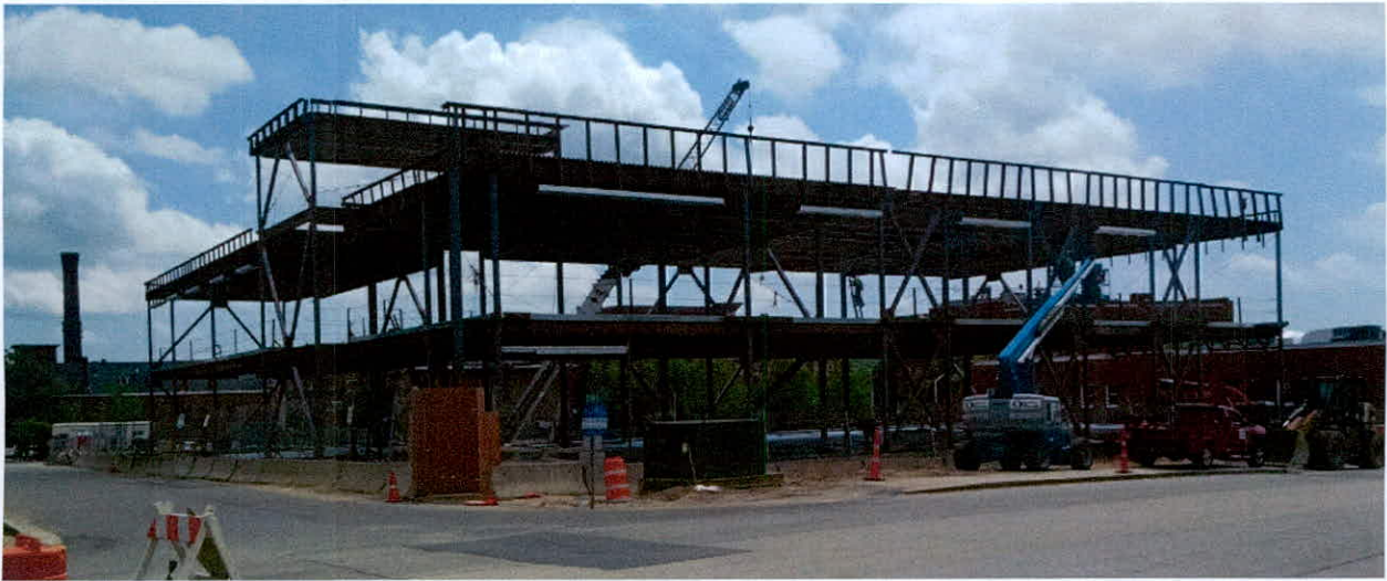
Steel Structure of police building – July 2015.
