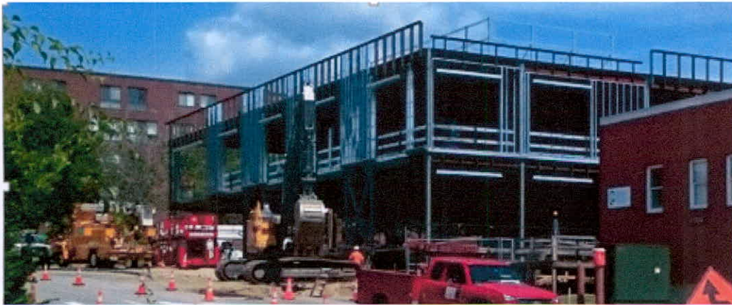
West façade of police building – August 2015.
