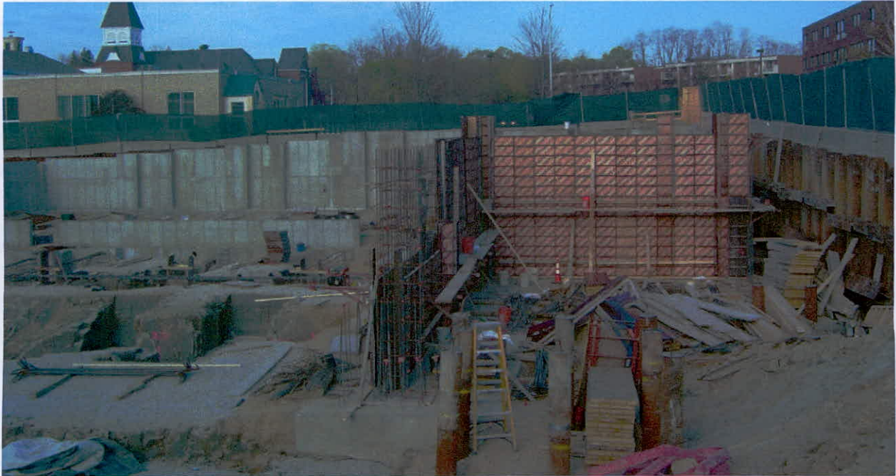
Construction of a foundation wall of the police Building – May 2015.
