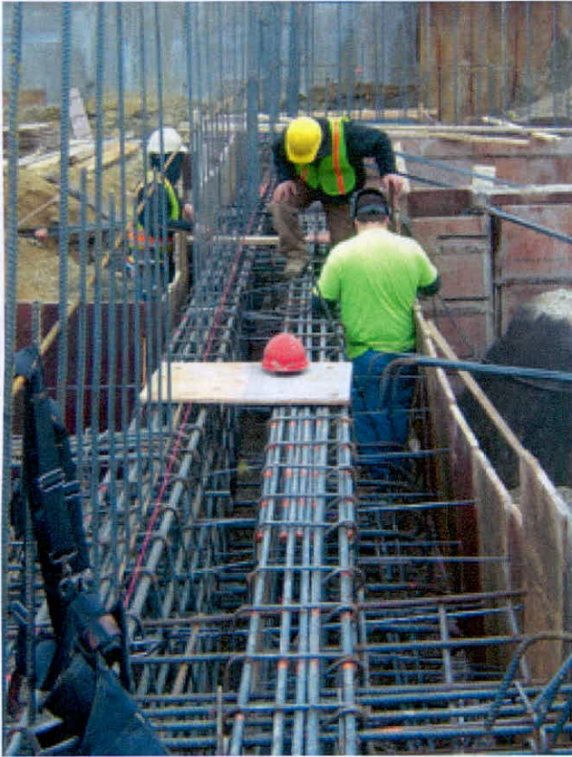
Installation of footing prior to concrete placement – April 2015.
