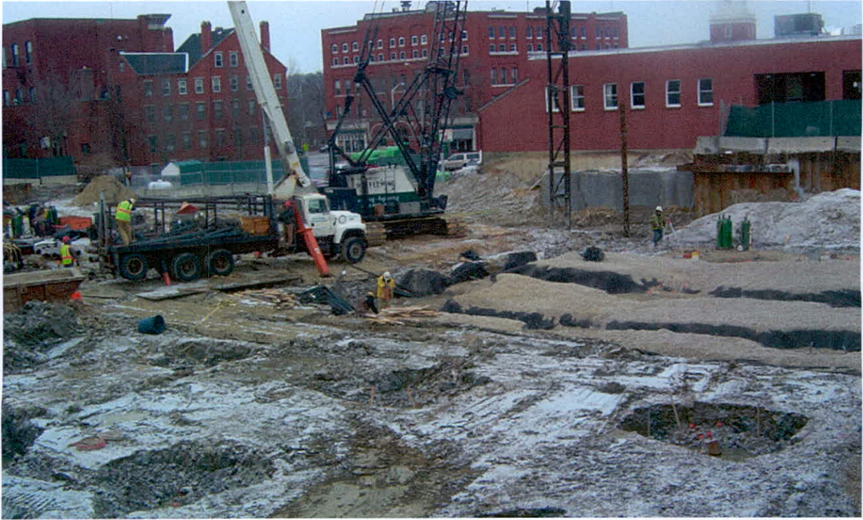
Installation of Building Support Piles – April 2015.
