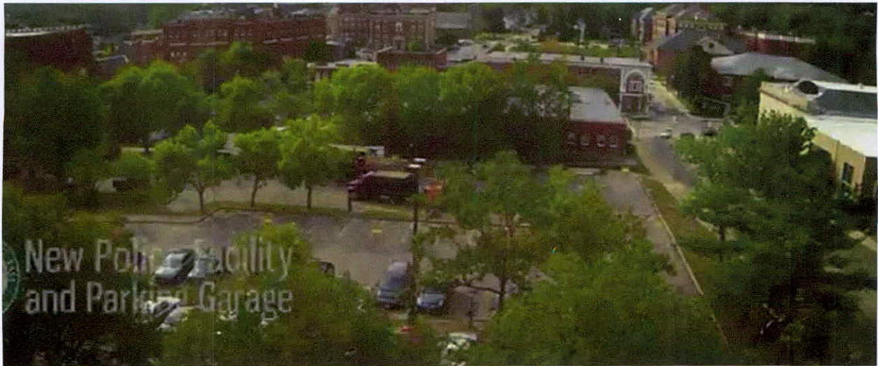
Orchard Street Parking Lot prior to the beginning of Construction – September 2014.
