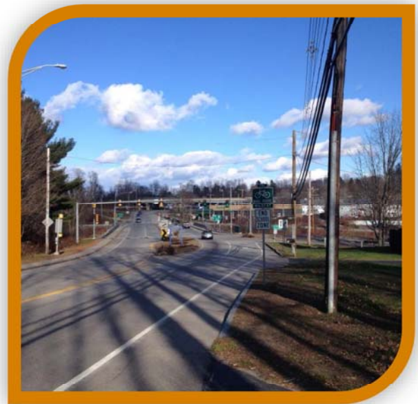
Route 108 at Back River Road
