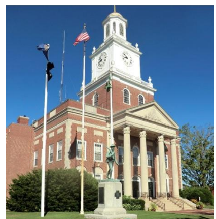
The Dover 2023 Vision seeks to integrate the City’s historic character with goals for creating a safe and inviting environment.
