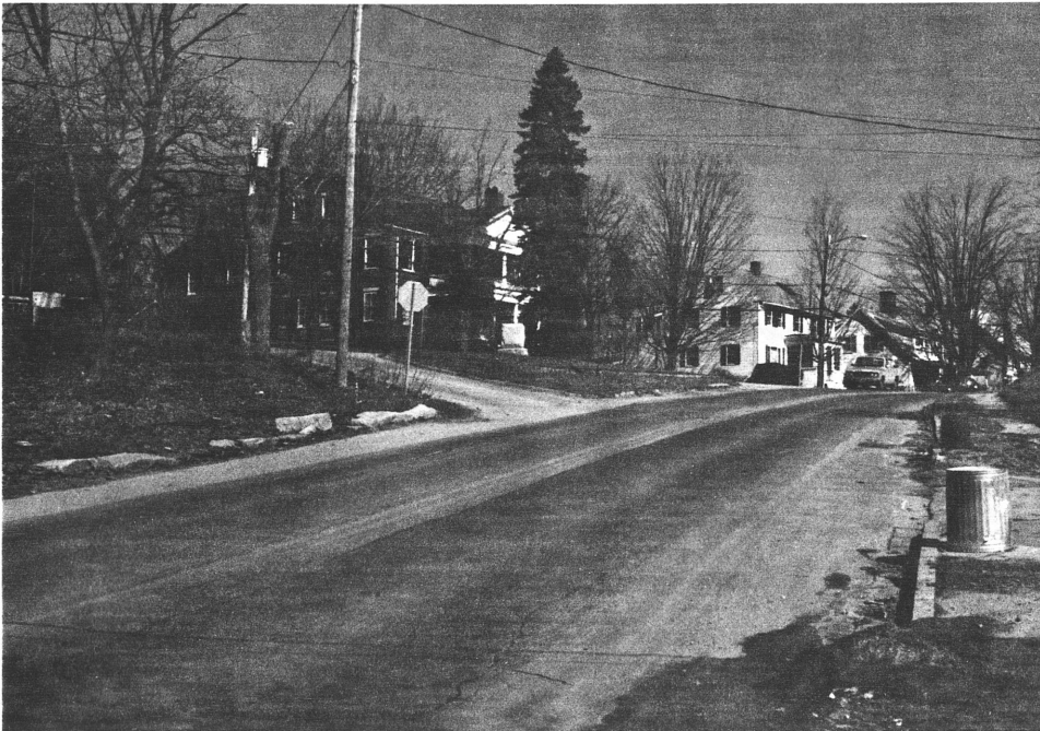
Portland Street Approach To Intersection
