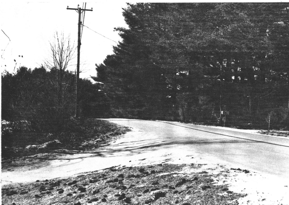
Drivers View Looking West Along County Farm Road At Intersection
