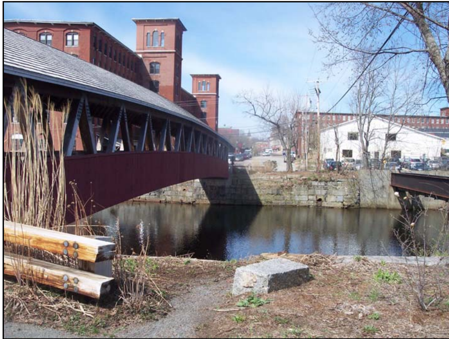
SUBJECT PROPERTY – FUTURE LOCATION OF WASHINGTON STREET BRIDGE Looking West - (4/07)
