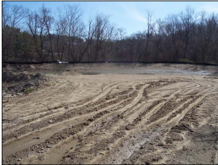
SUBJECT PROPERTY – NORTHEASTERN BURIED WASTE REMOVAL AREA Looking Northeast - (4/07)
