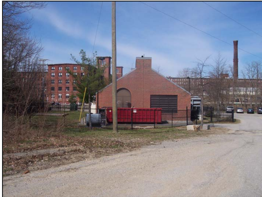
SUBJECT PROPERTY – THE WASTE WATER PUMP BUILDING Looking West from the future location of Washington Street - (4/07)
