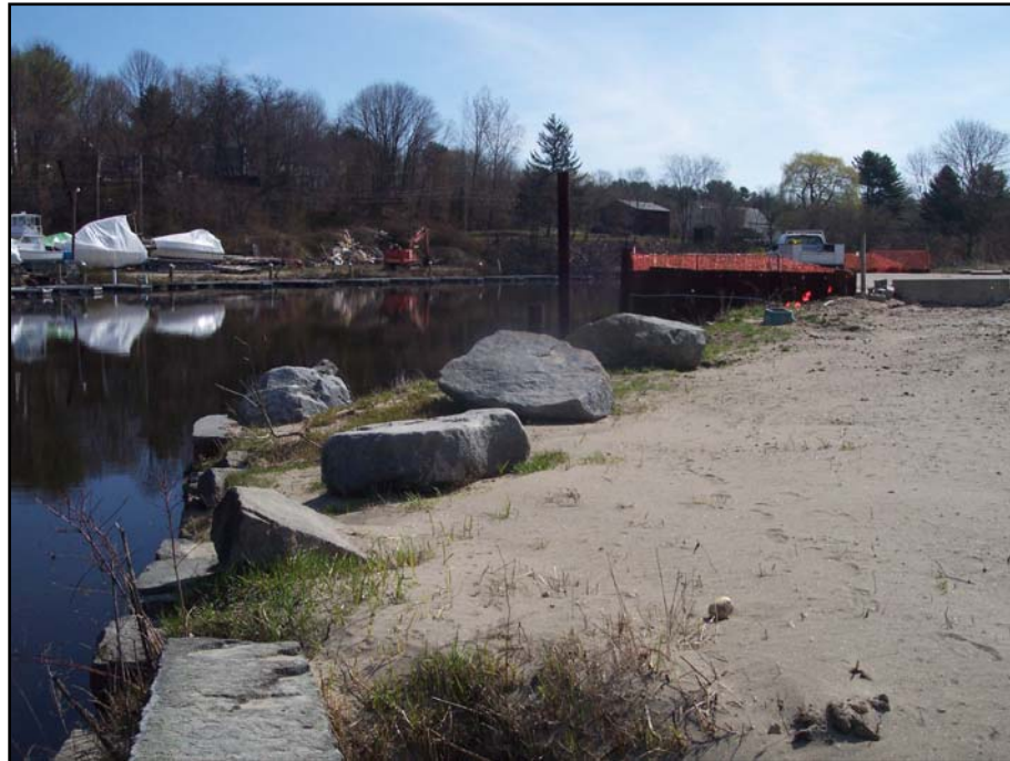
SUBJECT PROPERTY – FUTURE LOCATION OF THE PIER Looking Northeast along the Cocheco River - (4/07)
