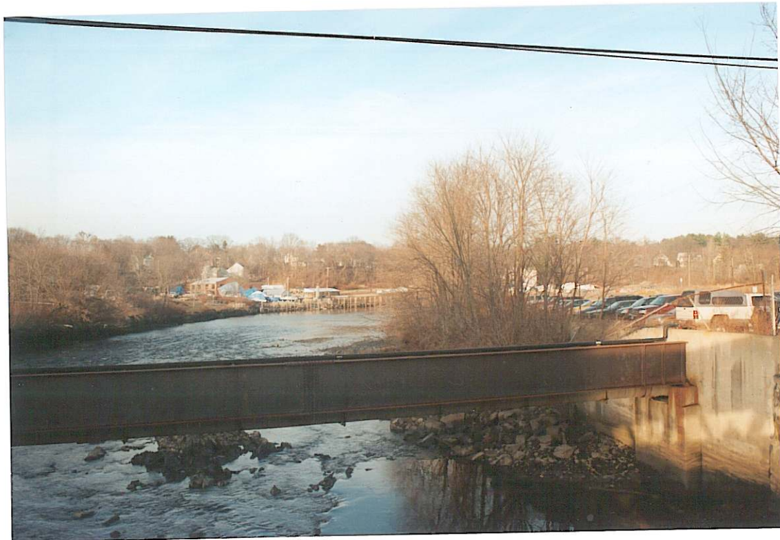
Another view of the Cocheco River this time looking north. The bridge in the foreground carries utility lines.
