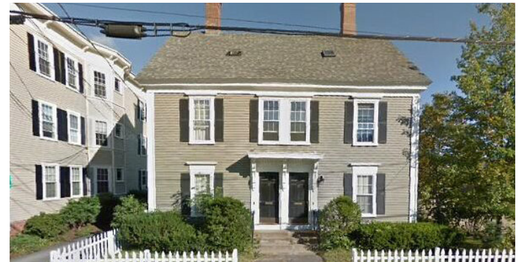
Kirkland Street Duplex, 11-13 Kirkland St.
