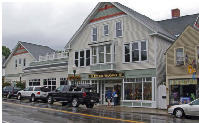
Larger gables flank this roof deck to provide elevated outdoor space.
