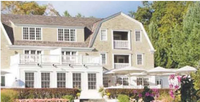
Example of small frontage building to screen mass and significant breaks in overall volume.
