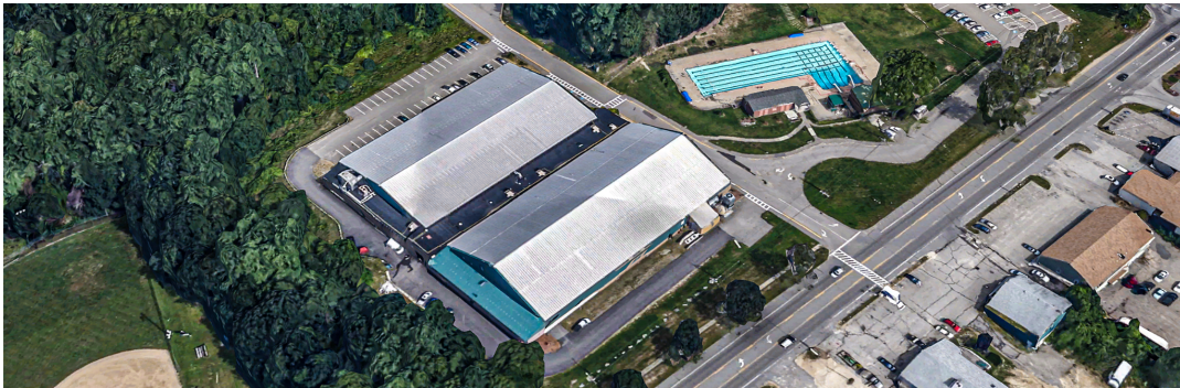
North up view of the Dover Ice Arena on Portland Avenue. Google Earth
